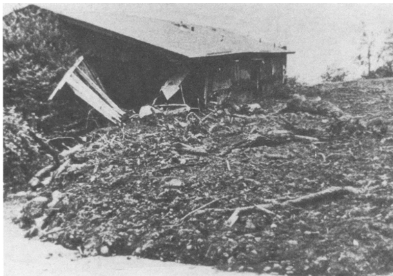
FIG. 5. Mudflow Frontal Deposit (Courtesy of USDA Soil Conservation Service, Salt Lake City)
