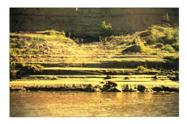
Figure 2.24 Erosion Generated by Wind Waves
