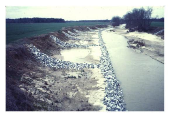
Figure 7.11 Longitudinal Stone Fill Toe Protection Riverward of High Bank With Tiebacks
