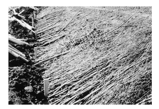
**Figure 27a**. Laying down the brush (basal end first) into a previously dug trench marked by row of wedge-shaped stakes.
