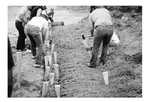
**Figure 27c**. Stretching the woven wire tight and securing by wedge-shaped stakes. Also, the wattling bundles are then laid over the top of the basal ends of the willow in the trench and secured tightly with wedge-shaped stakes.
