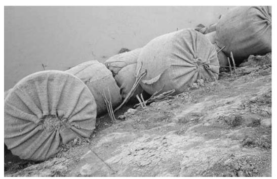
**Figure 10.** Vegetation in the form of dormant willow posts (discussed later) was placed landward of the rock and haybale toe.
