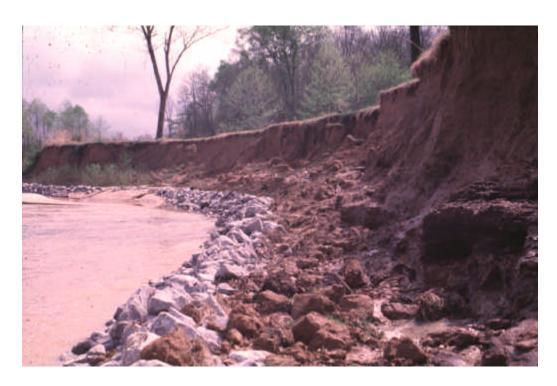
(a) One Ton Per Foot Immediately After Construction
