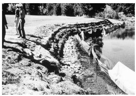
**Figure 32.** Vegetative geogrid during construction on the Upper Truckee River, California, near South Lake Tahoe. Note rock toe that was keyed into channel bed and bank to prevent undercutting. Photo was taken in October 1993.
