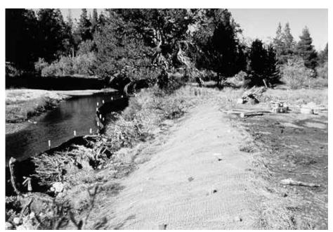
**Figure 38.** Burlap and coir woven fabric laid over sedge and grass seed, Upper Truckee River, California. Note that the fabrics were keyed in at the top and bottom in trenches and securely staked with wedge-shaped stakes. (Photo courtesy of Interfluve, Inc.)
