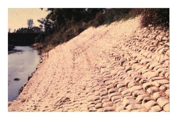
Figure 7.12 Typical Sack Revetment
