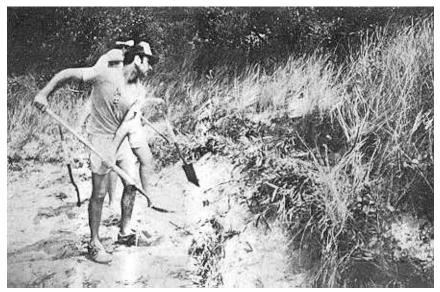
**Figure 29.** Installed section of brush layering. Note that brush has leaves because of a workshop setting. Normally, the brush would be without leaves because of installation during the dormant season.
