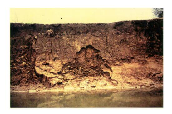
Figure 2.30 Pop-out Failure
