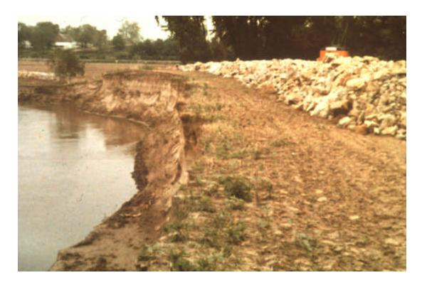
Figure 7.4 Conventional Windrow Placed on Top Bank
