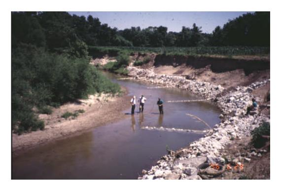
(b) Bendway Weirs in Combination with Longitudinal Peaked Stone Toe Protection
