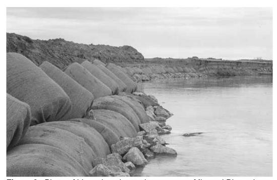
**Figure 9.** Photo of bioengineering project on upper Missouri River where large rock (1.5 Tons/lin ft) was used as toe protection below large coircovered haybales, also forming part of the toe.
