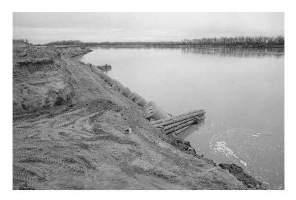
**Figure 3**. Timber cribs serving as deflection structures on the upper Missouri River to direct current away from the bank where there are bioengineering treatments.
