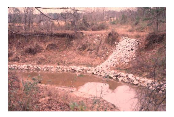
Figure 7.8 Typical Longitudinal Peaked Stone Toe Protection With Tiebacks
