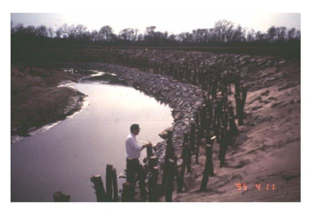
Figure 7.9 Longitudinal Peaked Stone Toe Protection In Combination With Willow Post Upper Bank Protection
