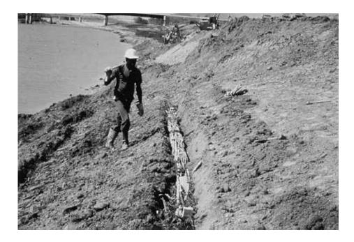
**Figure 39c.** Wattling (fascine) bundle being installed in the bank zone. Note that wattling should not be covered completely with soil; leave top 2-3" exposed for sprouting purposes. (Photo courtesy of Ms. Robin Sotir, Robin Sotir & Associates)
