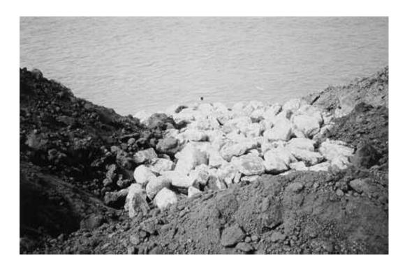
**Figure 4.** Rock refusal used on an upper Missouri River bioengineering project. Note that it is keyed back into the bank to prevent flanking of the upper and lower end sections of the project.
