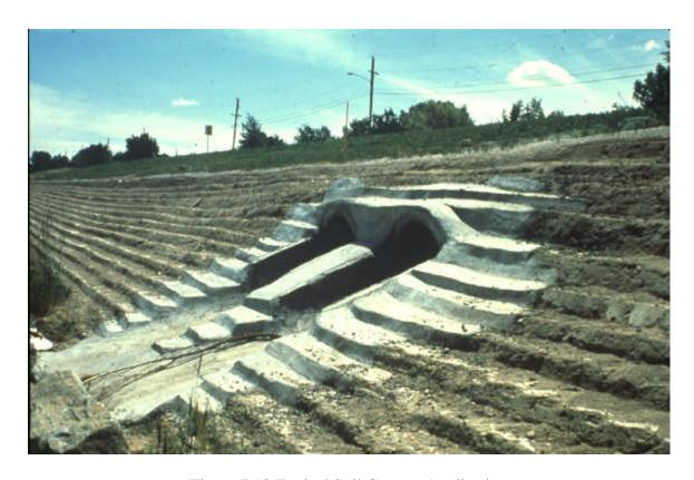
Figure 7.13 Typical Soil Cement Application
