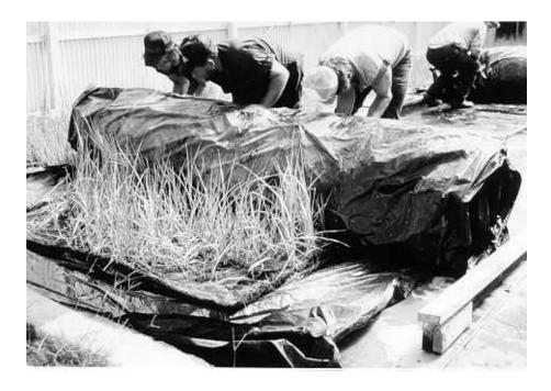
**Figure 25b**. Emergent aquatic plants established on a coir fiber mat being rolled up in the WES nursery ready for transport to the bioengineering site.
