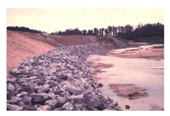
Figure 7.10 Longitudinal Stone Fill Toe Protection Placed Adjacent to Bank With Tiebacks
