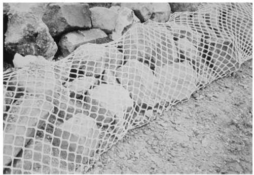
**Figure 11.** Rock roll used as toe protection on a bioengineering project, Rhine River, Germany, in the city of Dusseldorf.
