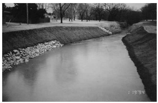
**Figure 8.** Photo of weighted rock toe revetment extending up the bank. It extends about 1/3 the distance up the bank. This photo shows the stream above low-flow conditions.
