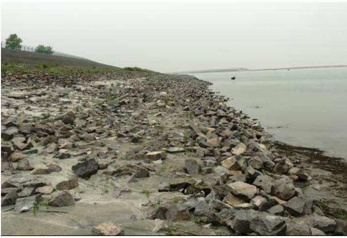
(a) Slope SP WGB below berm without damage
