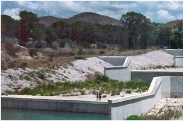
Figure 7-1 Gabion-armored threshold channel
