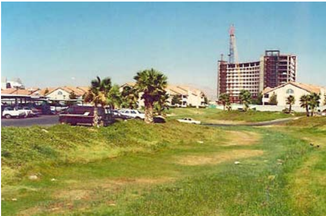
Figure 7-2 Grass-lined threshold channel
