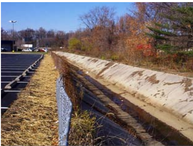
Figure 2-6 Stream encased by concrete channel
