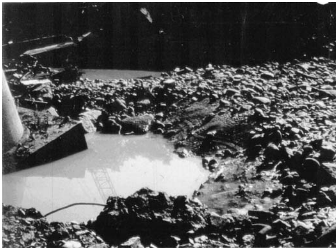
Note: Pier 2 is in the foreground with Pier 3 in the background.
