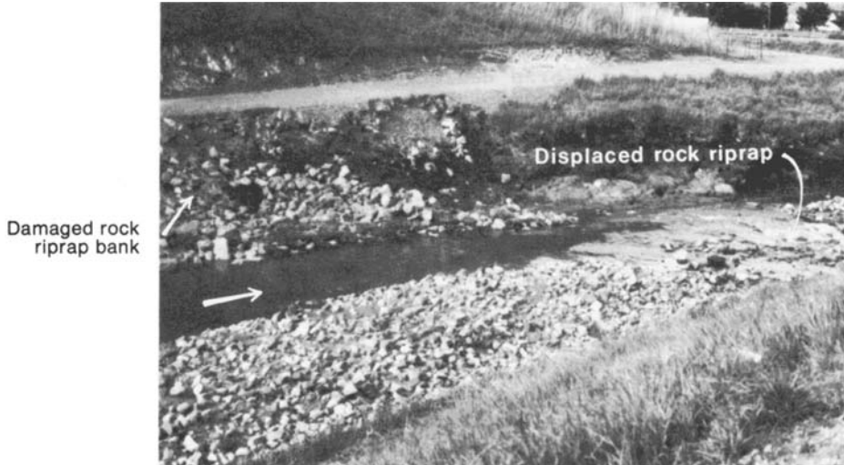
Note deposition of displaced riprap from upstream locations in channel bed (photographed March 1982). Source: Blodgett & McConaughy (1986)
