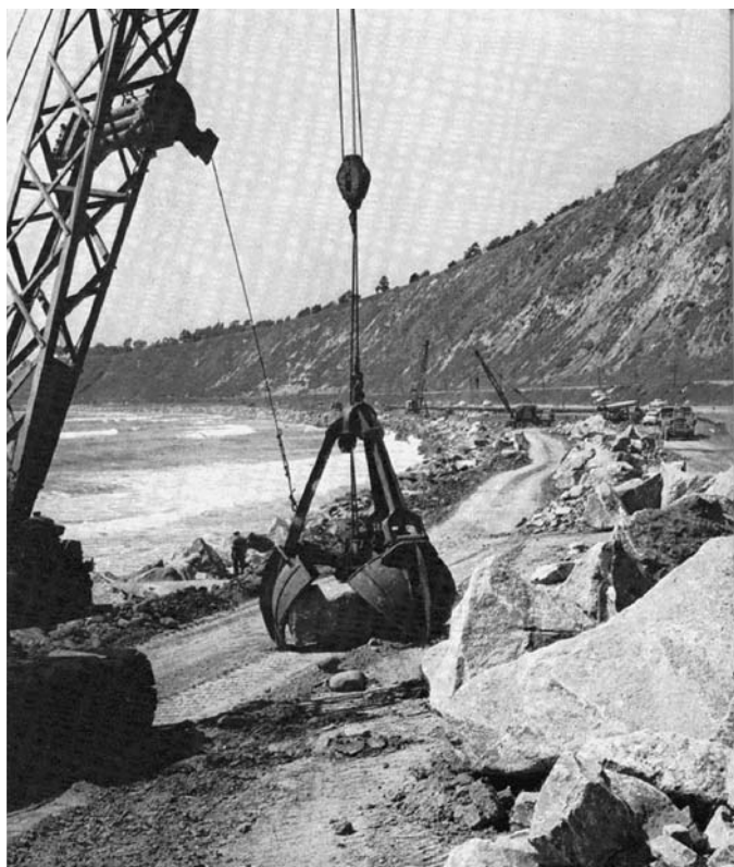
Figure 3.38. Orange-peel grapple picking up an individual large stone.
