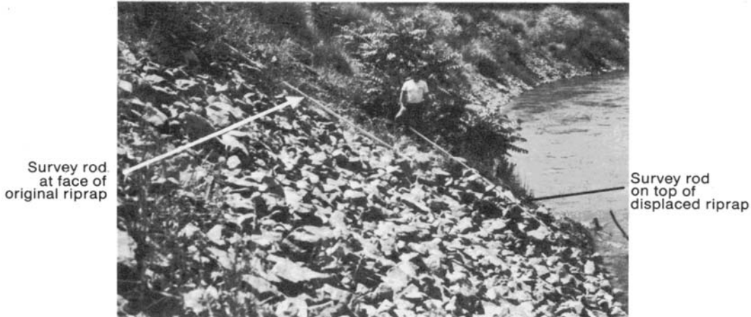
Figure D4.6. Riprap on Consumnes River at Site 3 near Sloughouse, California, looking downstream, showing modified slump failure (photographed May 31, 1983).
