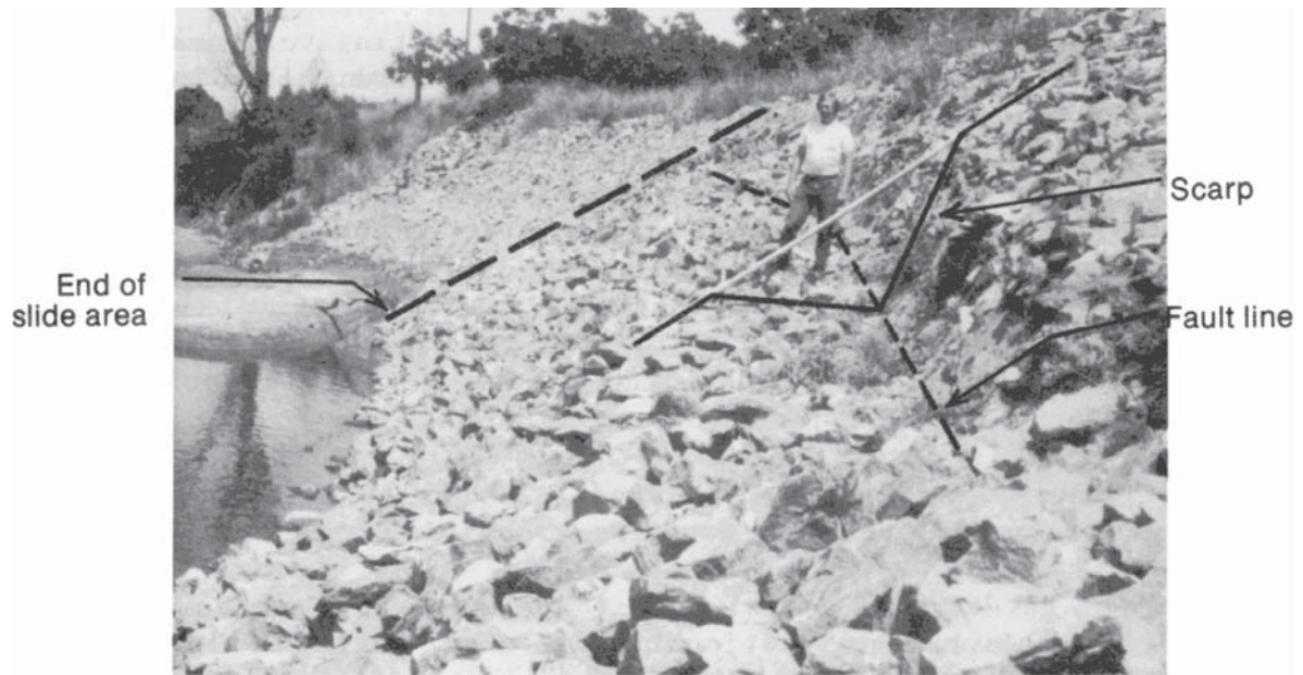
Figure 3.71. Riprap on Cosumnes River at Site 2 near Sloughhouse, California, looking down stream, showing translational slide failure (photographed May 31, 1983).
