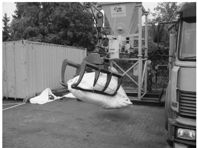
Figure 3.21. Handling a 1-tonne sand-filled geotextile, NCHRP Project 24-07(2).
