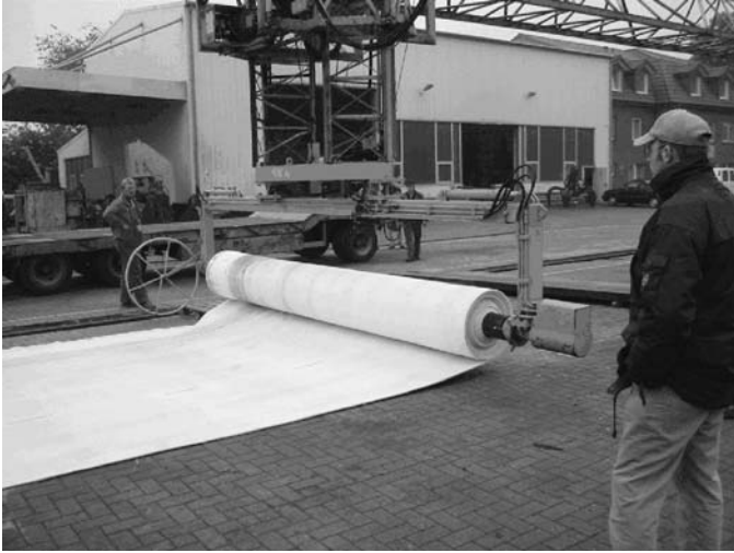
Figure 3.19. SandMat™ geocomposite blanket being unrolled, NCHRP Project 24-07(2).
