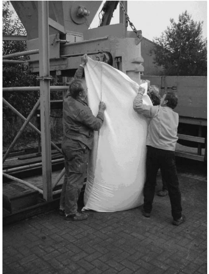
Figure 3.20. Filling geotextile with sand, NCHRP Project 24-07(2).
