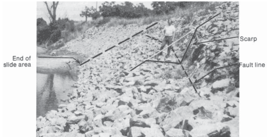
Figure D4.4. Riprap on Cosumnes River at Site 2 near Sloughouse, California, looking downstream, showing translational slide failure (photographed May 31, 1983).
