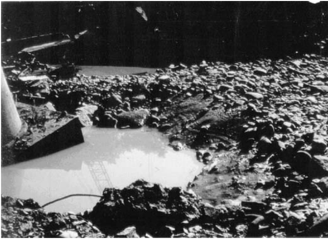
Pier 2 in the foreground with Pier 3 in the background.
