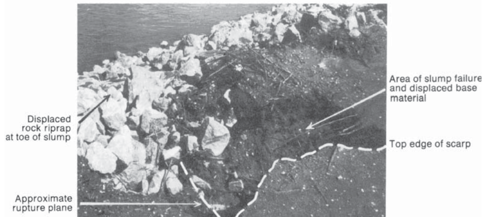
Figure 3.72. Riprap on left bank of Cosumnes River at Site 1 near Sloughhouse, California, showing slump failure (photographed May 31, 1983).
