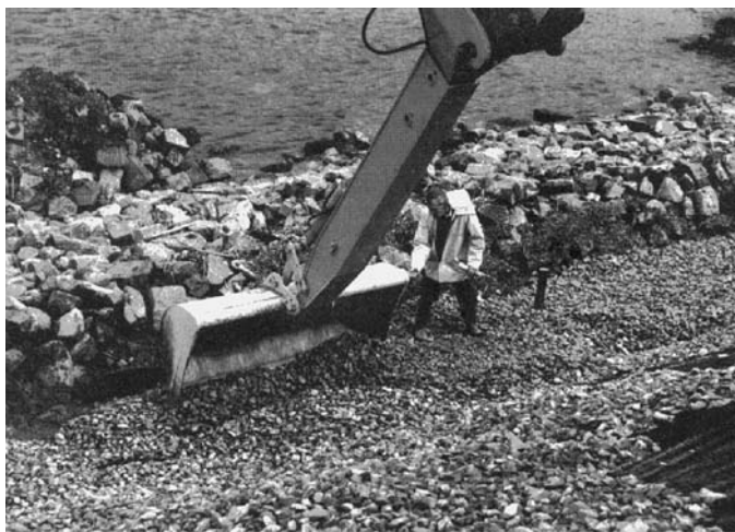
Figure 3.37. Slope trimming ahead of riprap placement.
