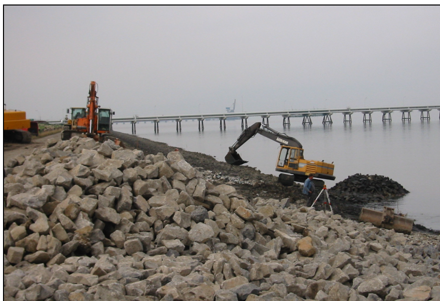
Figure 4.11. Placing riprap with hydraulic excavators.
