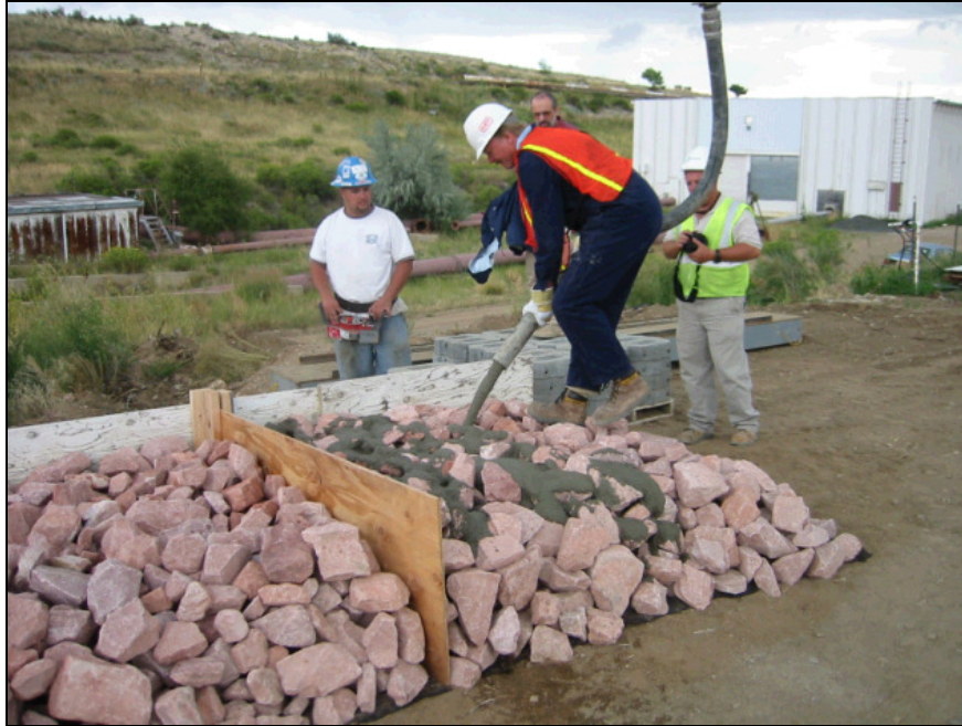
Figure 12.8. Preliminary trial grout application in the dry.
