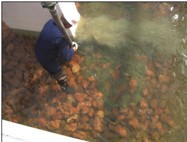
Figure 12.11. Underwater partial grouting of riprap.
