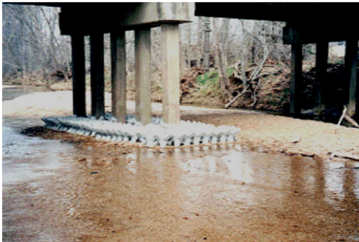
Figure 19.5b. Newly-installed A-Jacks armor units at Bridge 133, Graves County, KY
