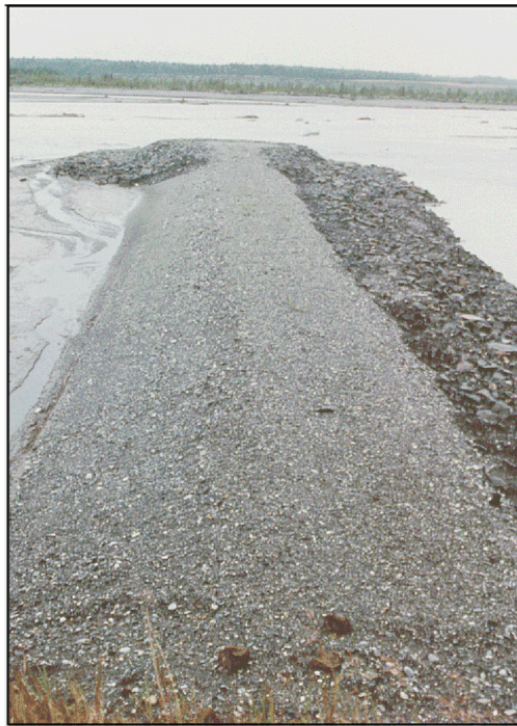
Figure 2.13. Impermeable spur field in top photograph with close-up shot of one spur in the lower photograph, vicinity of the Richardson Highway, Delta River, Alaska.
