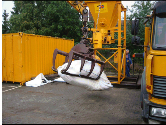
Figure 11.20. Handling a one-tonne sand-filled geotextile container. (photo from NCHRP Project 24-07(2), courtesy Colcrete – Von Essen Inc.)
