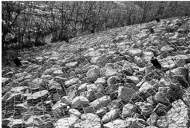
Figure 6.2. Wire enclosed riprap used for guide bank side slope protection at I-25 crossing of Rio Galisteo, New Mexico (NMSHTD).
