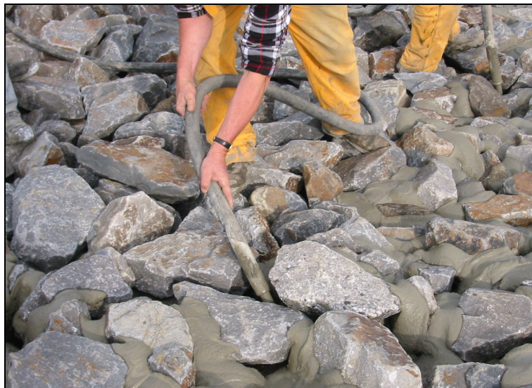
Figure 12.20. Grout placement by hand.
