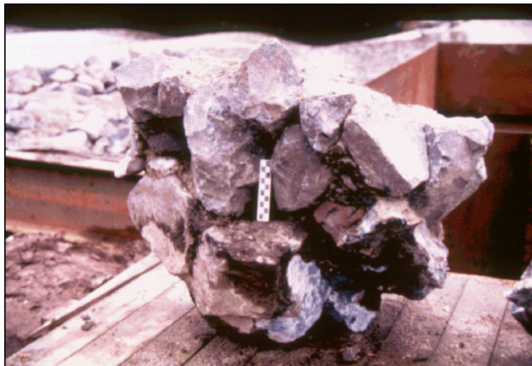
Figure 12.19. Conglomerate produced by spot grouting.
