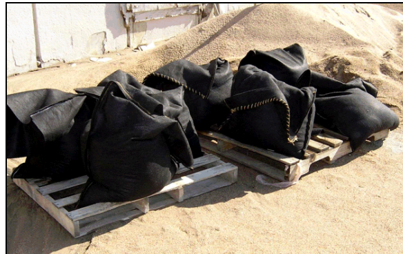
Figure 11.10. Geotextile containers before installation around the pier.
