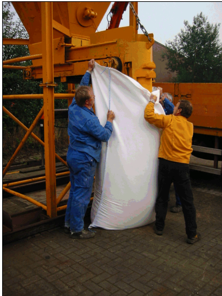
Figure 11.19. Filling geotextile container with sand. (photo from NCHRP Project 24-07(2), courtesy Colcrete – Von Essen Inc.)
