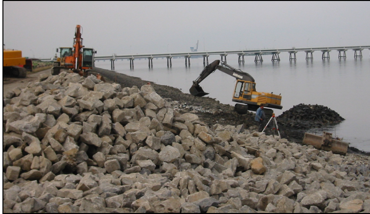
Figure 12.18. Placing riprap with hydraulic excavators.
