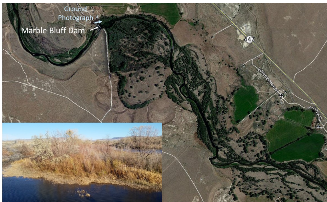
Figure A-2.—Vegetation has grown on extensive reservoir sedimentation behind Marble Bluff Dam, which is located on the Truckee River approximately 3 miles upstream from Pyramid Lake and 50 miles downstream of Reno, Nevada. The inset ground photograph is looking upstream at vegetated island that has formed on reservoir sediment deposit just upstream from the dam. The low-flow channel path is to the right of the island in this photograph, and a side channel has formed on the left side of the island. Aerial photograph is from Google Earth. The ground photograph was taken by Jennifer Bountry, Reclamation, November 18, 2016.
