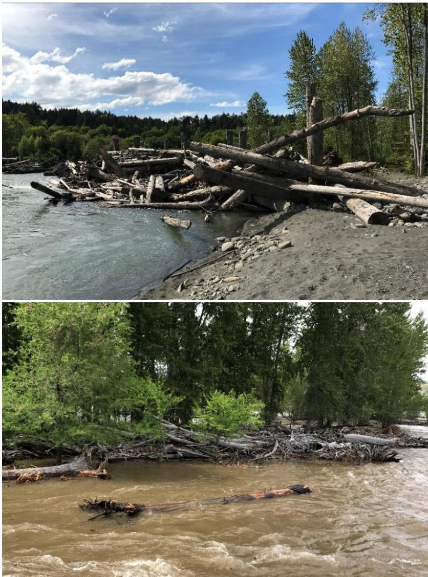
**Figure 8.—Top: A pile-supported engineered log jam can increase water surface elevation immediately upstream, creating a pool for aquatic species, influencing the distribution of shear stress in Elwha River, Washington. Photo: Jennifer Bounry, Reclamation. Bottom: Large wood accumulation on a mid-channel island during spring runoff on the Methow River, Washington. Photo: Reclamation.**
