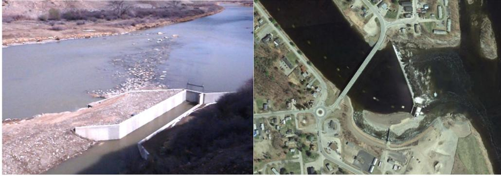
**Figure 15.—Left: A low-head diversion weir constructed from natural, non-grouted materials replaced a push-up dam on the North Fork of the Gunnison River, Colorado. It allows for fish and boater passage and provides a low-maintenance solution for water diversion. Right: A bypass channel constructed around Howland Dam, Maine, for migratory fishes. Photos: Jeff Crane, Crane and Associates, Inc. (left) and Google Earth (right).**
