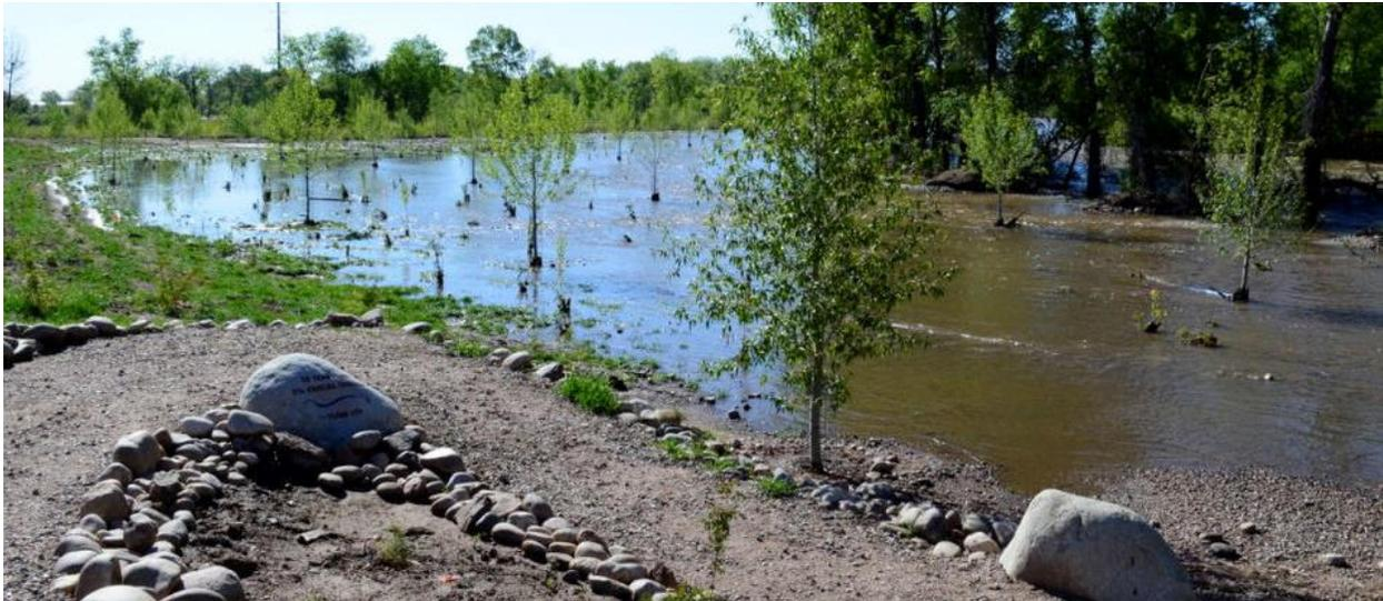
**Figure 7.—Example of a floodplain rehabilitation on the Poudre River, Fort Collins, Colorado. A levee was removed and a floodplain bench excavated and re-vegetated to hydrologically connect with the incised river. Gravel quarries adjacent to the river were also reclaimed and connected with flood flow paths. Photo: Joel Sholtes, Reclamation.**
