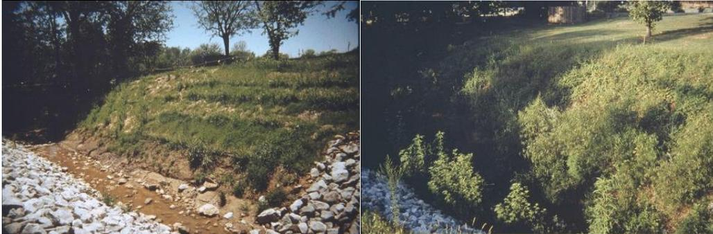
**Figure 11.—Example of streambank bioengineering (right side of pictures) with riprapped bank (left side of pictures) in first year of construction (left) and two years later (right). Credit: Natural Resources Conservation Service.**
