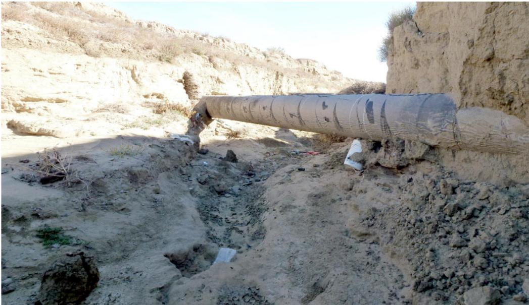
**Figure 9.—Formerly buried pipeline exposed by gully incision (note headcut in lower left) in a desert wash, Navajo Reservation, New Mexico. Photo: Michael Sixta, Reclamation.**
