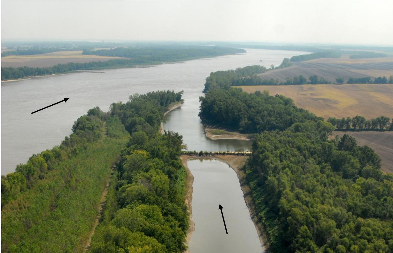
FIGURE 5.13 Looking downstream at closure dike on secondary channel on Mississippi River. Note widened bankline just below the dike caused by the plunge pool when the dike is overtopped.
