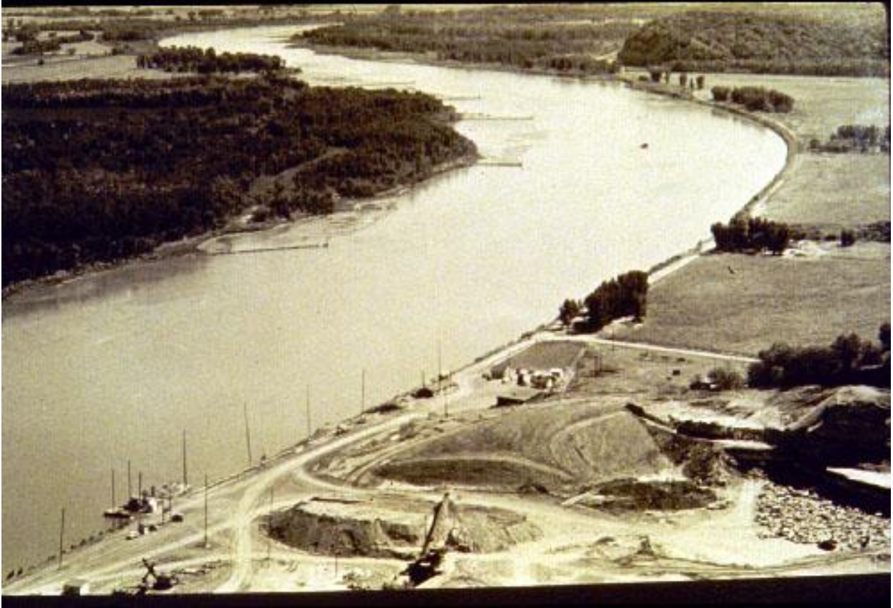
FIGURE 5.23 Rock Bluff Bend, Missouri River, 1956
