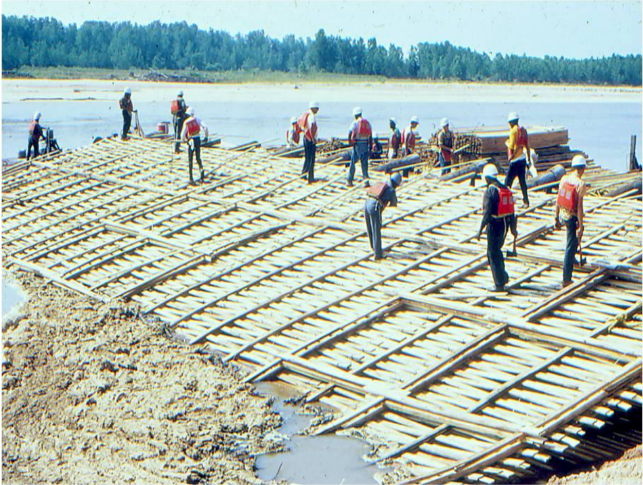
FIGURE 6.3 Section of board mattress revetment under construction
