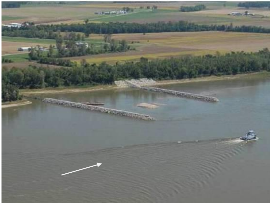
FIGURE 5.7 Dike Bank Paving On The Upper Mississippi River
