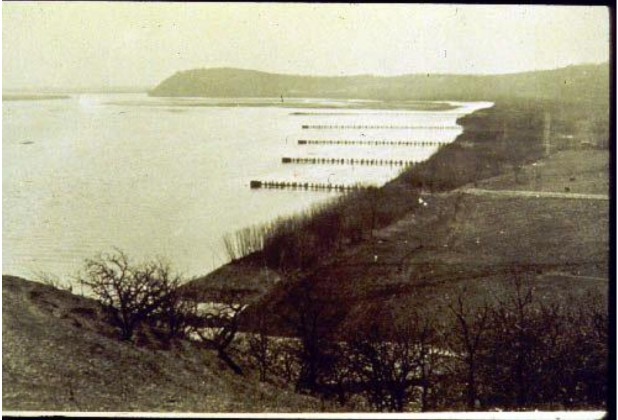
FIGURE 5.20 Rock Bluff Bend, Missouri River with Timber Pile Dikes, March 1935
