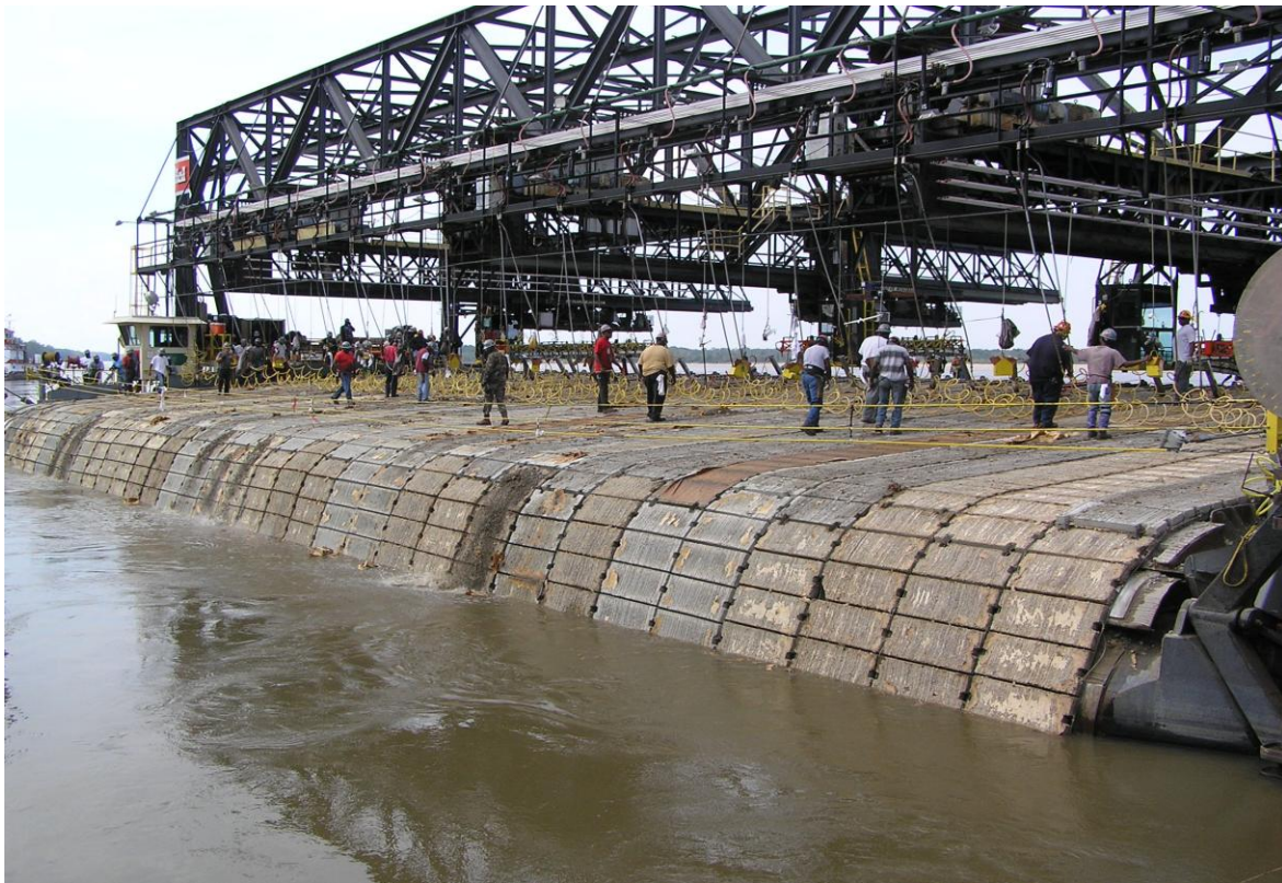
FIGURE 6.5 ACM Revetment Schematic and Sinking Photograph
