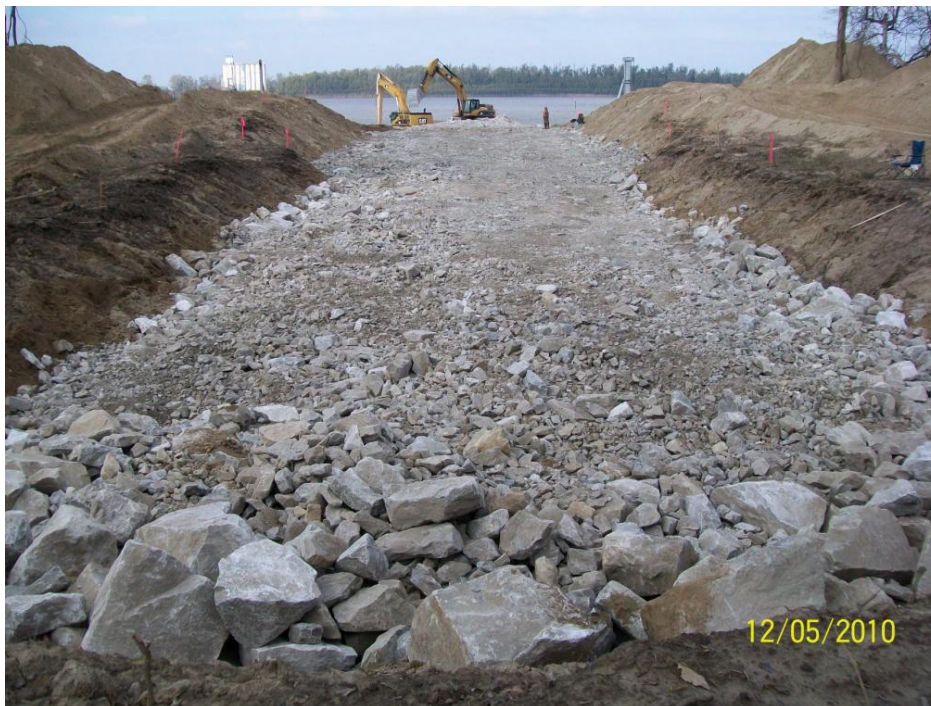
FIGURE 5.6 Stone Placed In Stone Root On The Mississippi River
