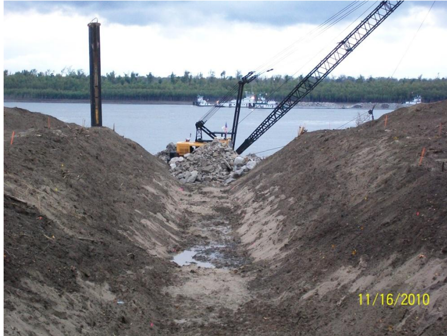
FIGURE 5.5 Excavated Trench For Stone Root On The Mississippi River
