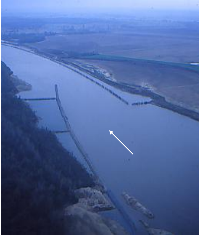
FIGURE 5.14 Crain Revetment Kicker Dike, Red River. Louisiana
