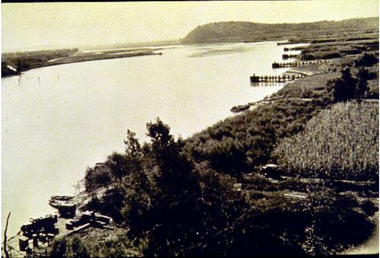
FIGURE 5.21 Rock Bluff Bend, Missouri River Showing Deposition in Timber Pile Dike Field, October 1939
