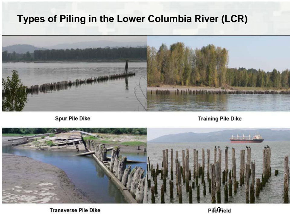
FIGURE 12,1 Types of pile structures on the lower Columbia River channel
