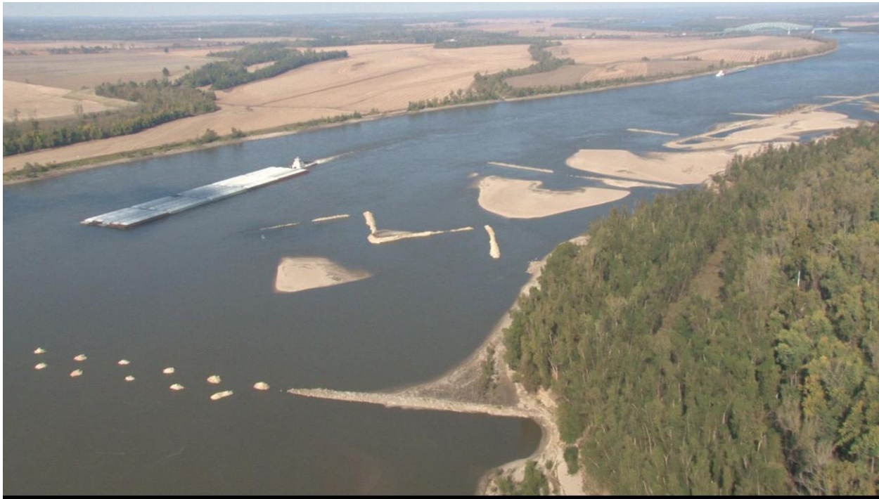
FIGURE 1.1 Photograph showing the use of dikes and revetments on the Mississippi River
