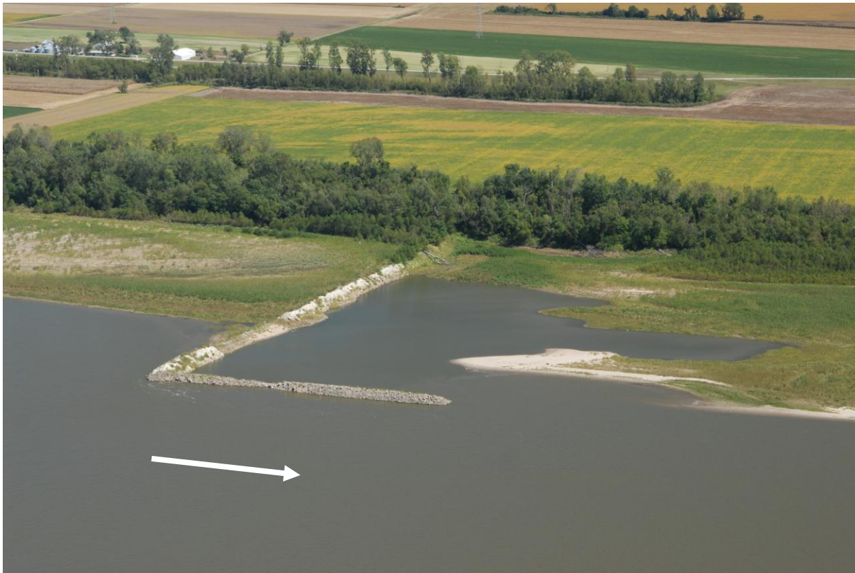
FIGURE 5.12 L-head dike on the Mississippi River
