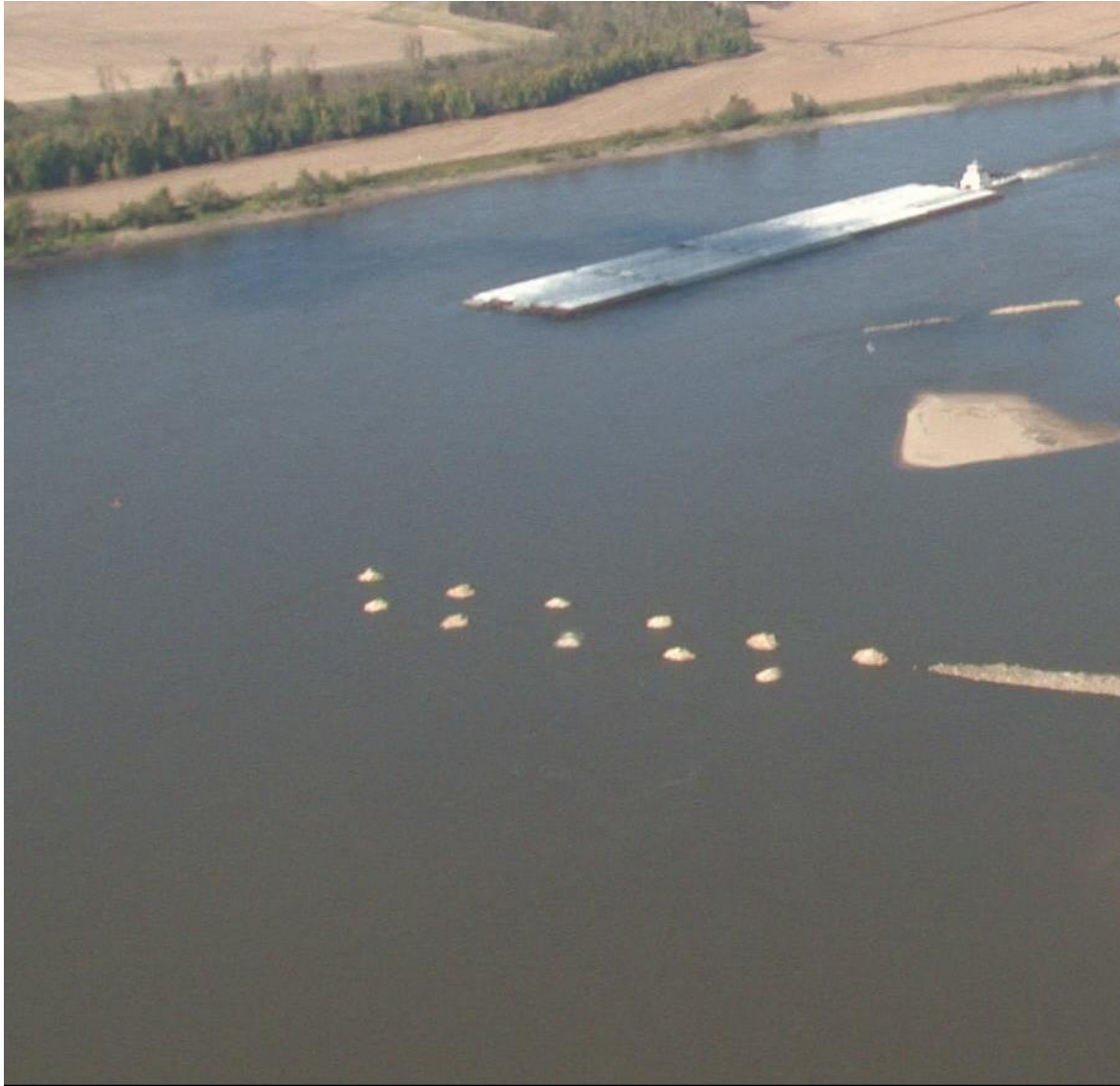
FIGURE 10.2 A double row of Multiple Roundpoint Structures on the Mississippi River, St. Louis District
