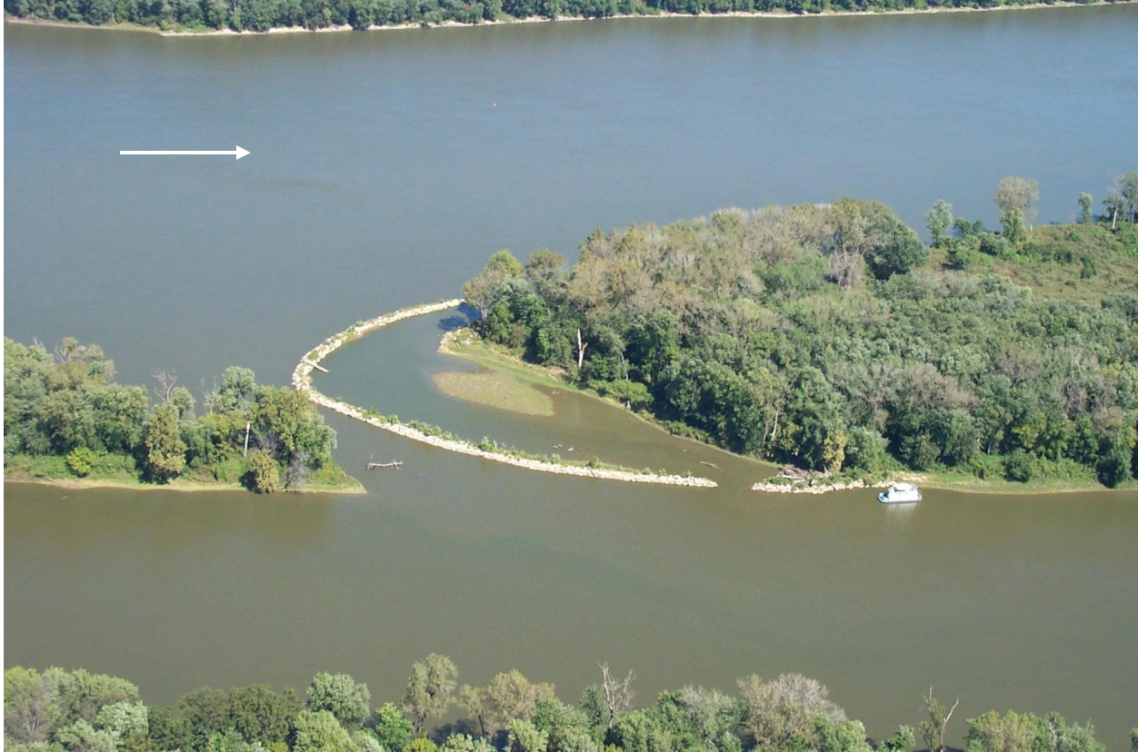
FIGURE 7.4 Photograph of bullnose structure on Mississippi River
