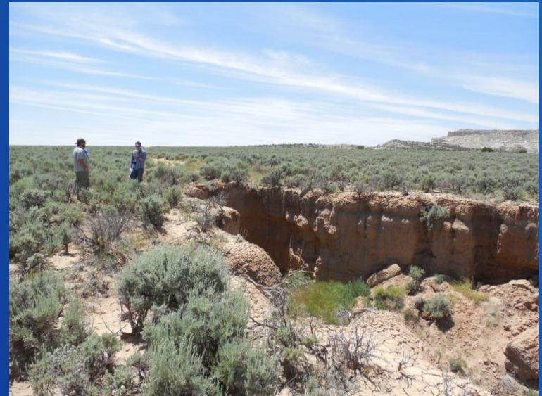
25 to 30 ft. deep head cut. Pipeline about 75 ft away.
