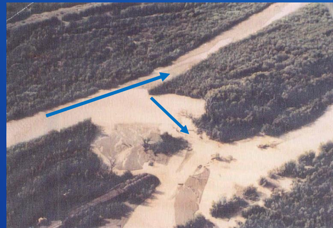
1991 Tiffany Levee Breach
