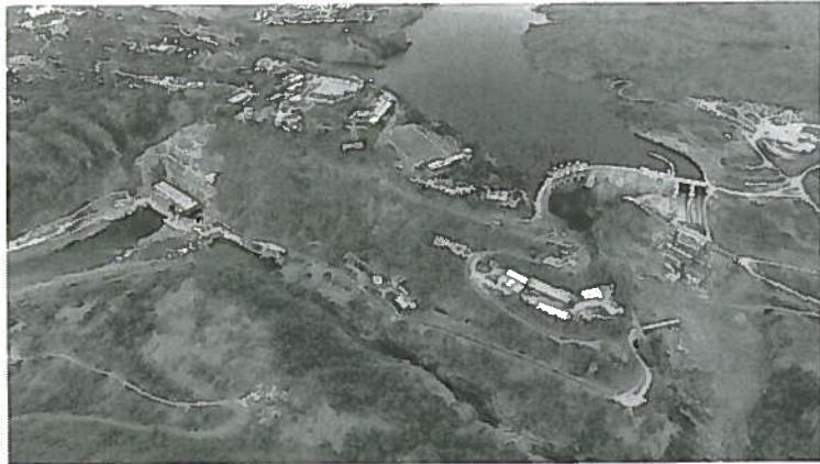
Figure 15. Aerial view of the completed Cambambe Dam
