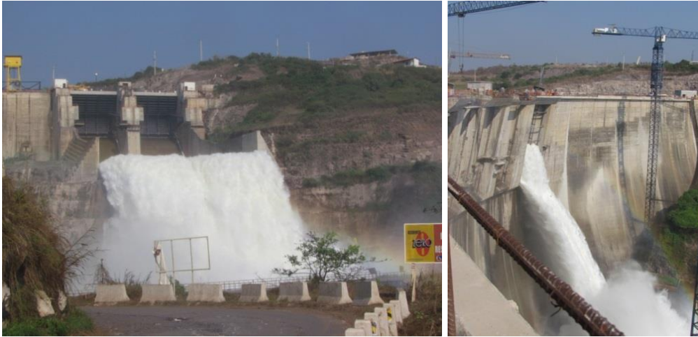
Figure 11: Spillway test in 2016
