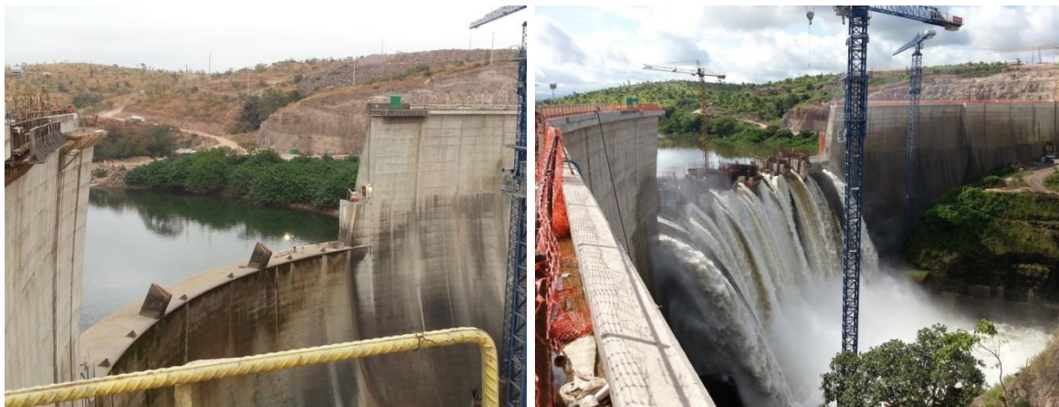
Figure 5: Pictures from the dam site during the dam heightening
