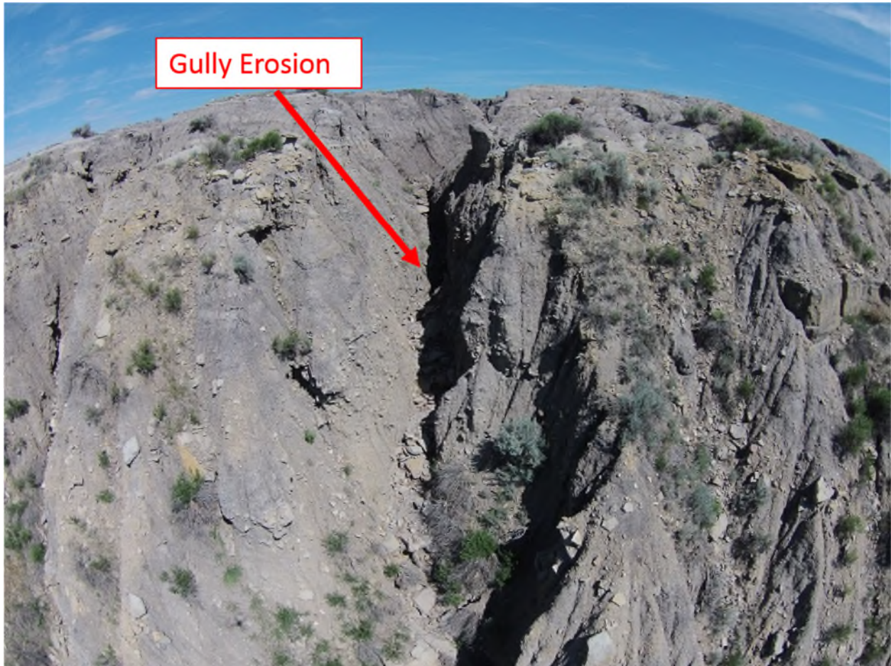
Figure 7 Example of Gully Erosion on Eastern Side of Bluff B at Riley Pass
