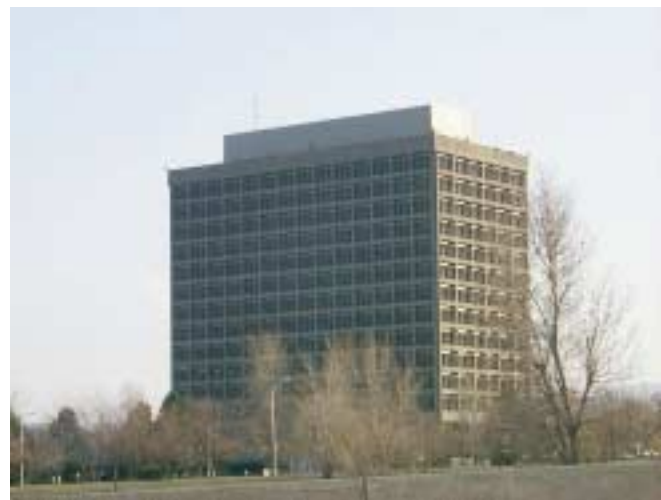
Fig. 1. Building 67, Denver Federal Center, CO
