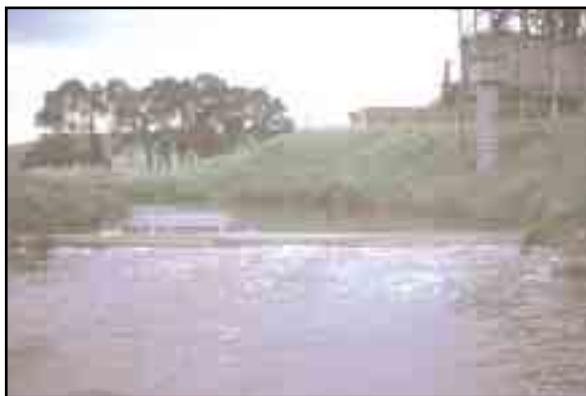
Figure 8.3. The weir for a gauging station on the Wando River, Victoria. Providing fish passage over this weir could reduce its accuracy as a gauge.
