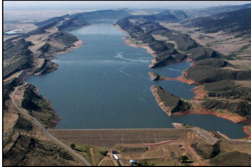
Fig. 1. Local example of an earthen dam. Aerial view of Horsetooth Reservoir looking south. Source: www.northernwater.org .
