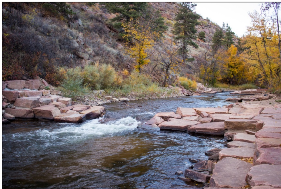
Figure 3.1. Photo of a WWP structure looking upstream during low discharge.
