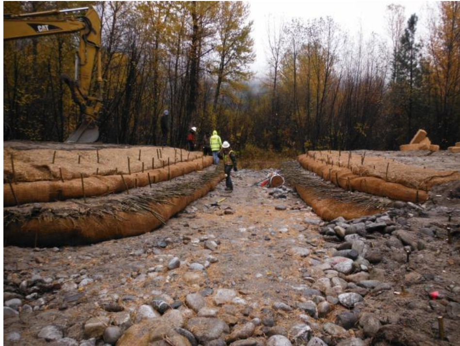
Photograph 12 Completed installation of FESL looking downstream
