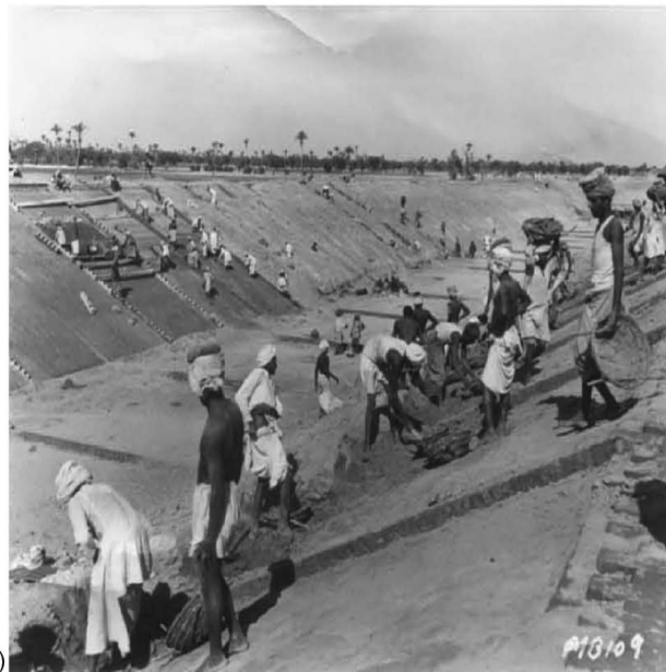
Fig. 10. Construction of the Link Canals in Pakistan with (a) heavy equipment; (b) extensive labor
