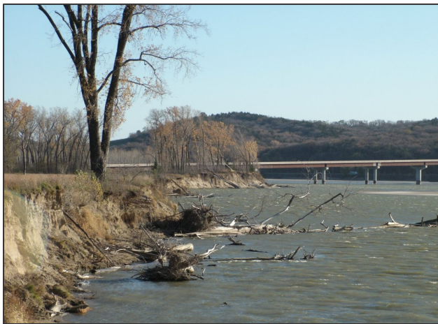
Missouri River at Well Field showing undercut banks
