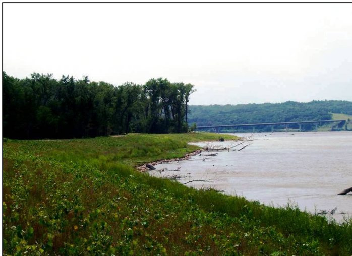
Completed Stabilization with locked logs, grass and young cottonwoods
