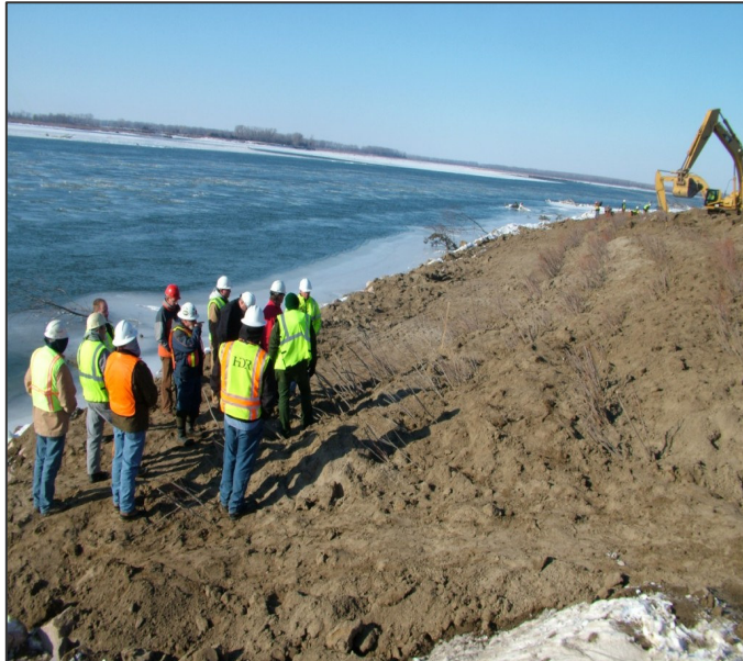
Partners discuss construction methods
