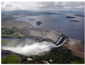
[Illustrated is flow in two of the three spillways of Guri Hydroelectric Project, Caroni River, Venezuela. The spillways have aeration ramps and flip buckets. This photo shows the resulting free-jet profile and the associated plunging jet. Note the use of concrete gravity and earthfill portions of the overall dam.]
