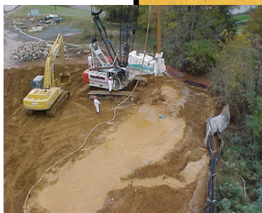
Top: Iron filings used to treat chlorinated solvents. Above: Deep soil mixing process. Left: DuPont's application of the ZVI-Clay
