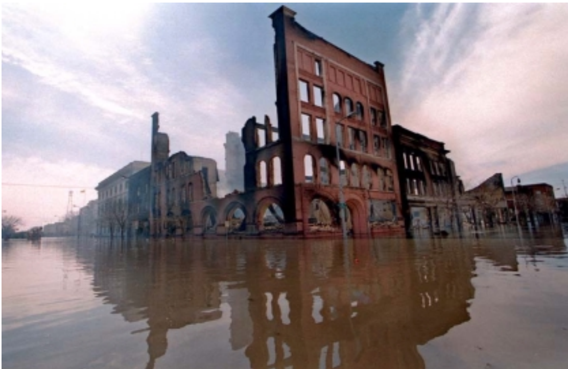
Figure 4. Downtown Grand Forks, North Dakota, after floodwaters from a once in 500-year flood ruptured a gas line, igniting a fire that claimed eleven office buildings. Photo by Eric Hylden, Grand Forks Herald.
