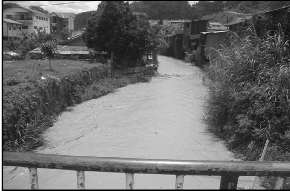
Figure 13: Water Level Gradually Increases Due to Restriction of Flow by Adjacent Structures and Bridge at CH 900
