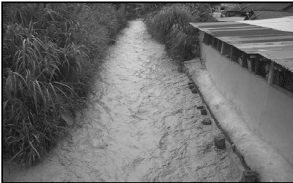
Figure 12: Water Level Seen Almost Breaching the Base Level of Building Nearby. Depth of Water Recorded at 0.8 m at Discharge of 4 m 3 /sec.
