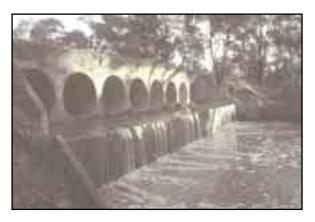
Figure 4.3. A culvert that could pose a barrier to fish passage.
