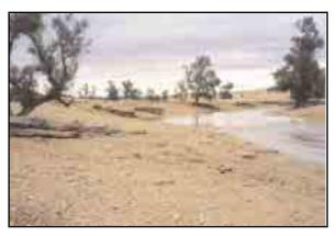
Figure 11.1. The impact of an over-enthusiastic contractor. This bank was meant to be only slightly battered, and the groynes should have been on the toe of the bank, protruding into the base flow.
