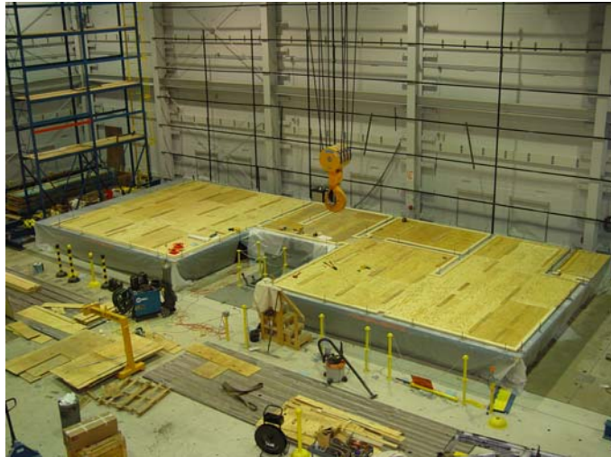
Fig 3 Construction of Foundation for NEESWood Benchmark Test Structure.
