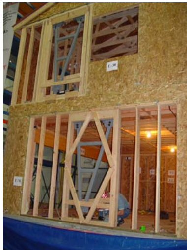
Modular Damper Wall Units installed in First and Second Story of Benchmark Structure
