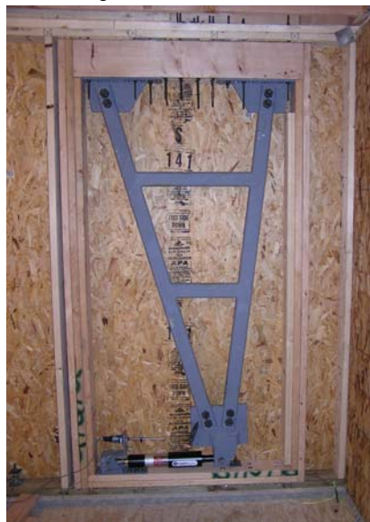
Modular Damper Wall Unit installed in Benchmark Structure (view from inside of garage)
