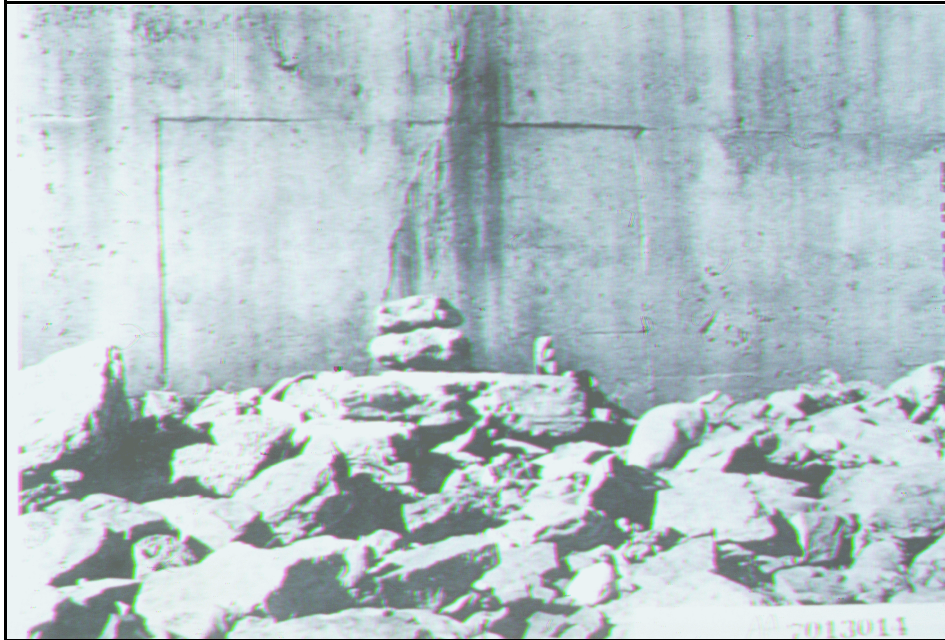
Figure 11.1. Photograph of riprap at pier 2, October 1956. (98,99)
