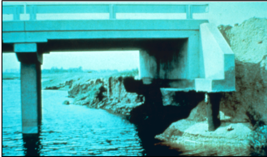
Figure 7.2. Scour of bridge abutment and approach embankment.
