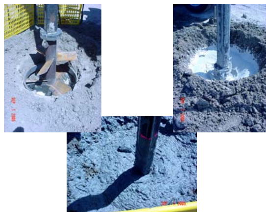
Mixing of 3-foot diameter test columns at the Suncor refinery
