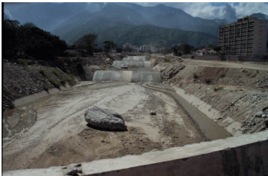
Figure 6.20: Control canal for debris flow at the Saint Julian Ravine, Leon and Rojas, 2000 (personal communication)
