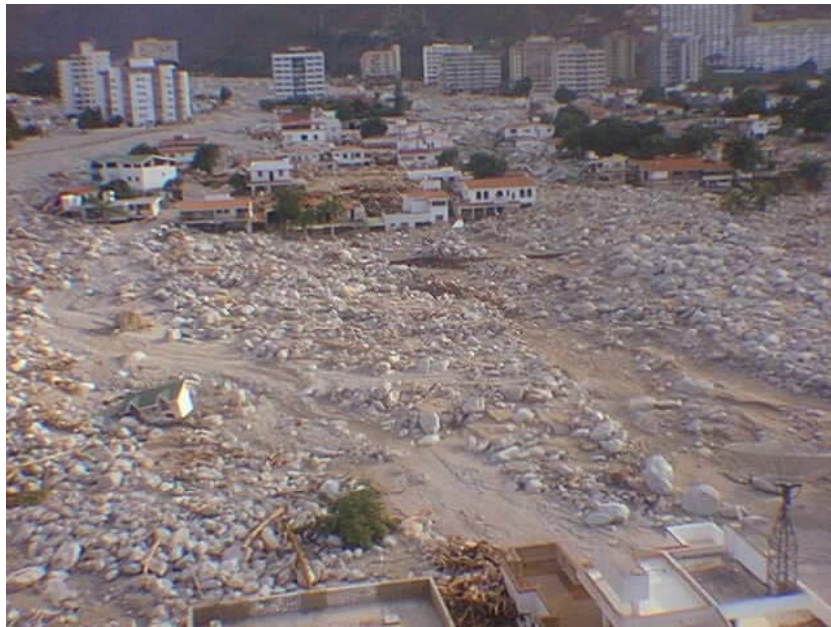
Figure 6.12: View of road damaged in Los Corales, Leon and Rojas, 2000 (personal communication)
