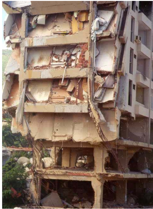
Figure 6.19: View of damaged to apartment building in Los Corales, Leon and Rojas, 2000 (personal communication)
