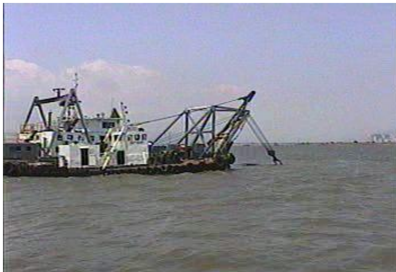
Figure 3-17. Sediment dredging on the Lower Nakdong River
