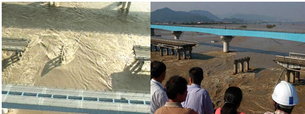
Figure 3-3. Gupo Bridge failure after Typhoon Maemi
