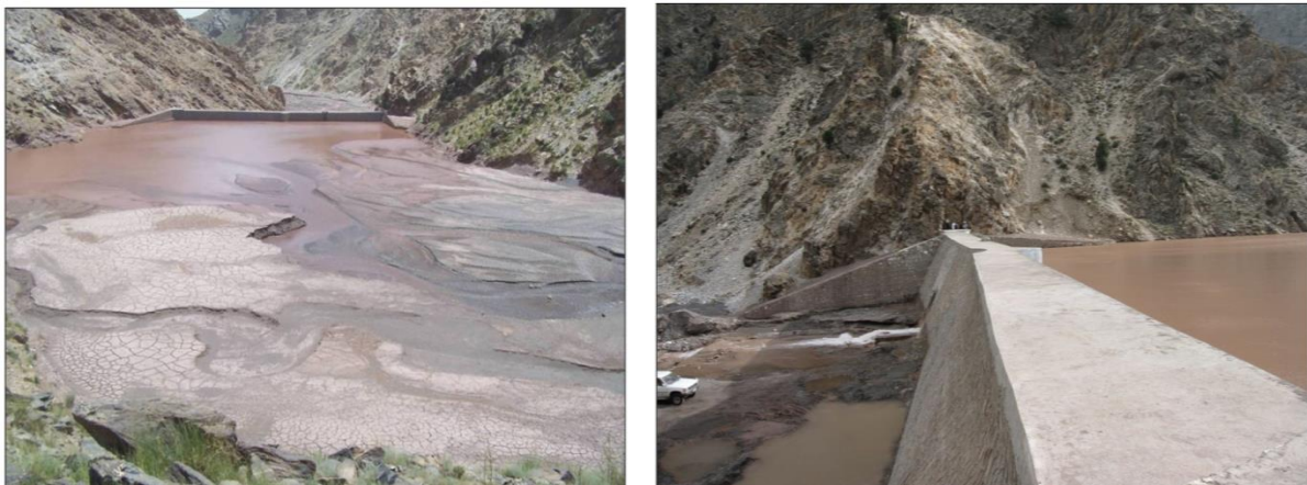
Figure 1.4 - Hezarak Dam, a) Upstream of the Filled Reservoir b) Along Top of the dam (USACE 2009)
