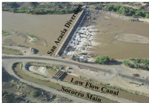
b) San Acacia Diversion Dam
