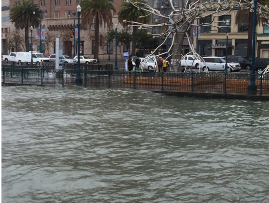
Figure 31 - San Francisco Bay waters overtopping the seawall and spilling onto the adjacent walkway immediately southeast of the Agricultural building November 24, 2015 (USACE 2016)
