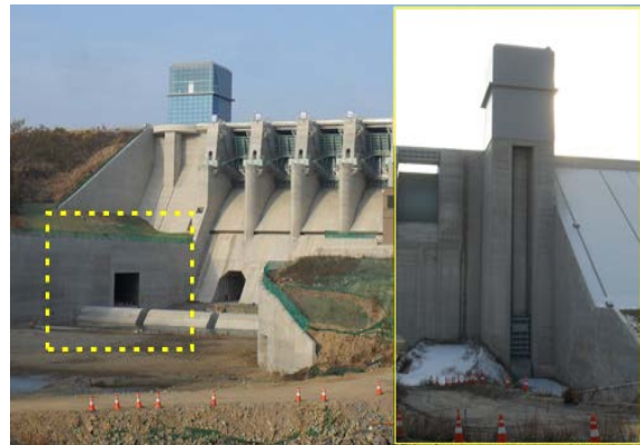
Figure 113: Photos of Yeongju multi-purpose dam facilities: intake tower (up), sediment detention reservoir constructed 13 km upstream from the main dam (middle), and sediment through installed on main dam (down)
