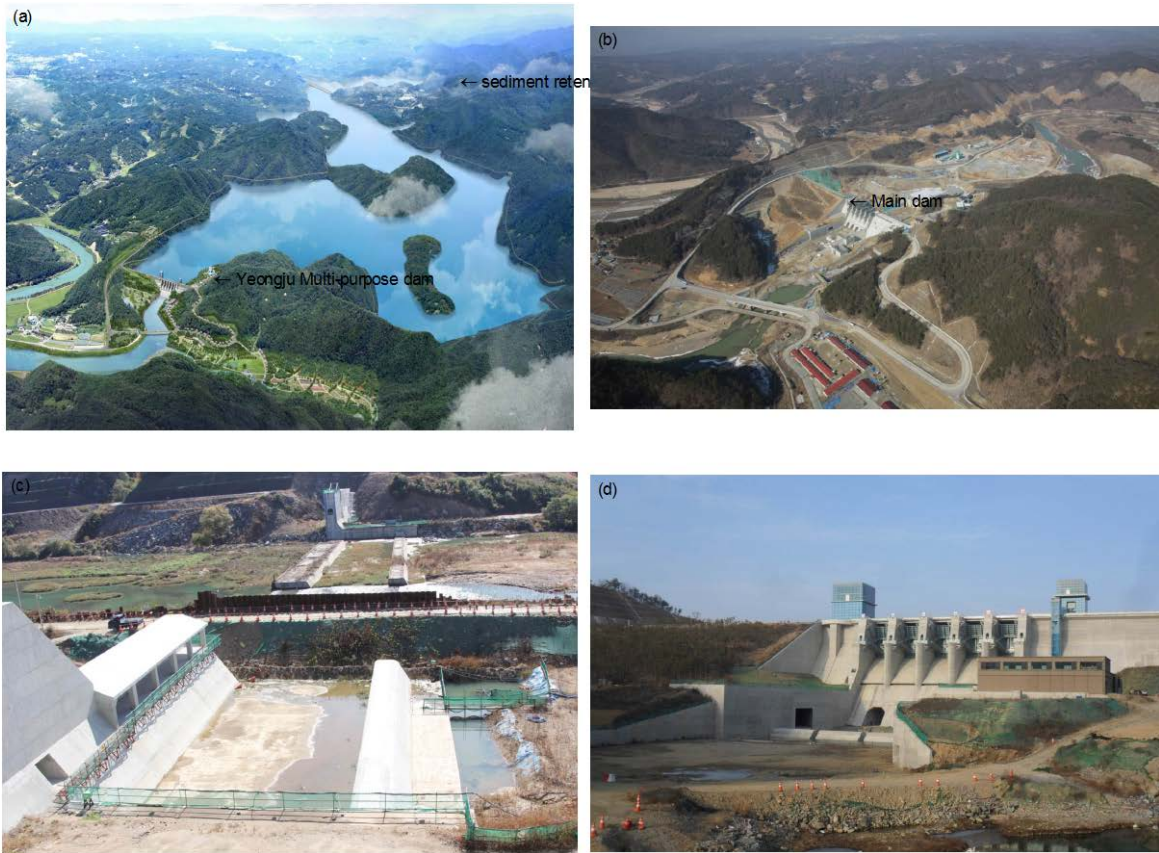
Figure 17: Sediment detention facility of Yeongju multi-purpose dam
