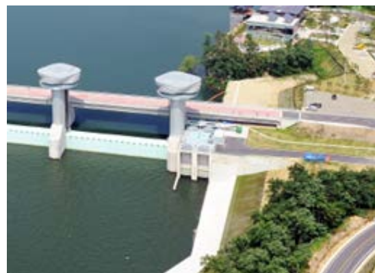
Figure 116: Photos of Sangju Weir facilities: shell type roller gates and flap gate (up) and hydropower plant (down)
