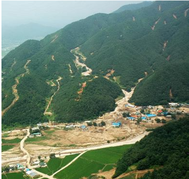
Figure 1.1. Damaged area in Inje County in Gangwon Province, South Korea
