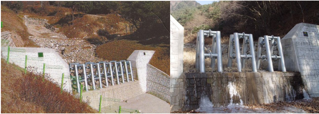
Figure A.3. Slit dam example in Duksan Creek
