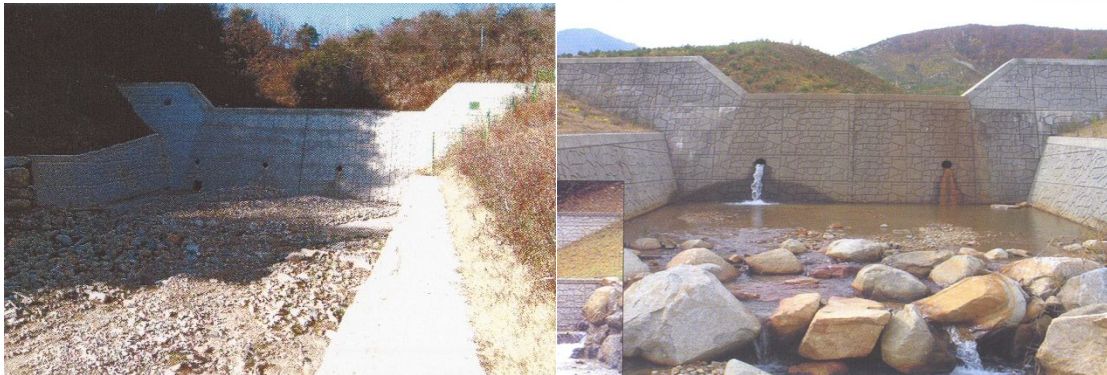
Figure A.5. Concrete dam example in Duksan Creek
