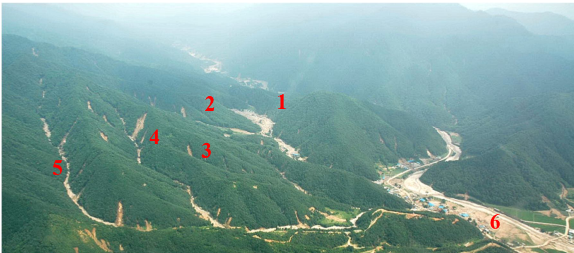
Figure 5.24. The comparison between shear stress and real damaged area
