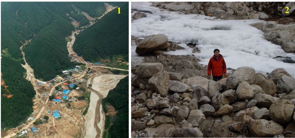
Figure 5.27. Damaged areas due to debris flows
