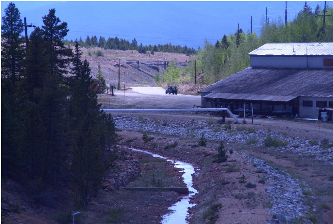
Figure C-10: View looking downstream at double channel in California Gulch near Yak Tunnel Portal below CG-1 gauge. Flow from the Yak Tunnel is collected from the left channel and delivered to the treatment plant approximately one-half mile downstream. Flow from the upper California Gulch (there is none in this photo) bypasses the treatment plant via the channel at right.
