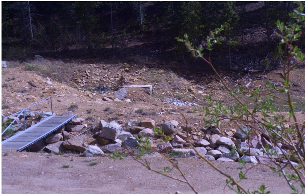
Figure C-8: Defunct flume adjacent to CG-1 and above Yak ditch. Bridge in foreground crosses the outflow channel below the CG-1 pool.
