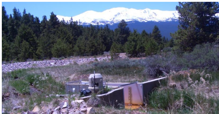
Figure 4.15: CG-5 with data-logger in case on left bank.
