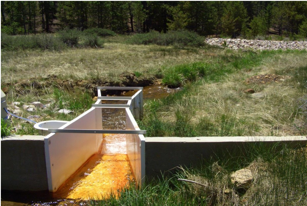
Figure C-36: CG-5 flume inlet and view downstream.
