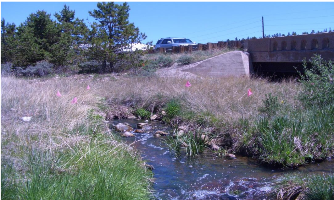
Figure C-46: WWTP discharge culvert downstream of US-24 bridge. Pink flags are CDOT wetland delineation.
