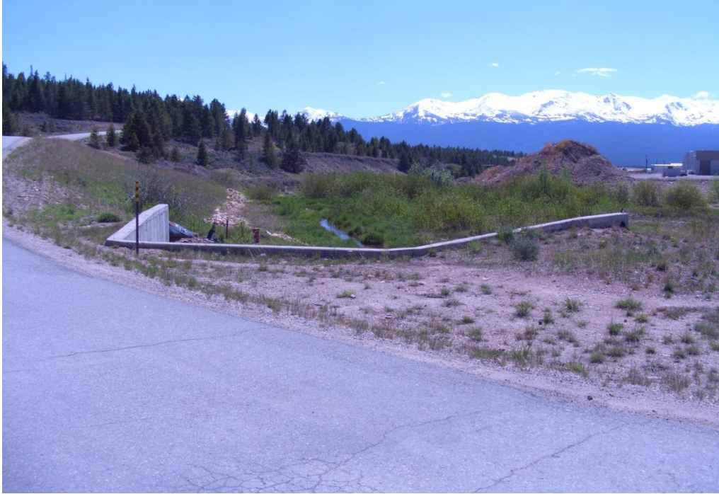
Figure C-15: View looking downstream (west) from County Road 6 bridge over California Gulch.
