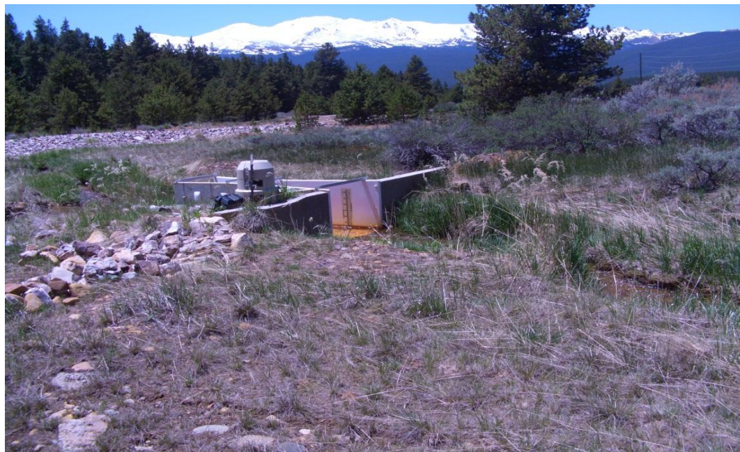
Figure C-38: CG-5 flume and surroundings.
