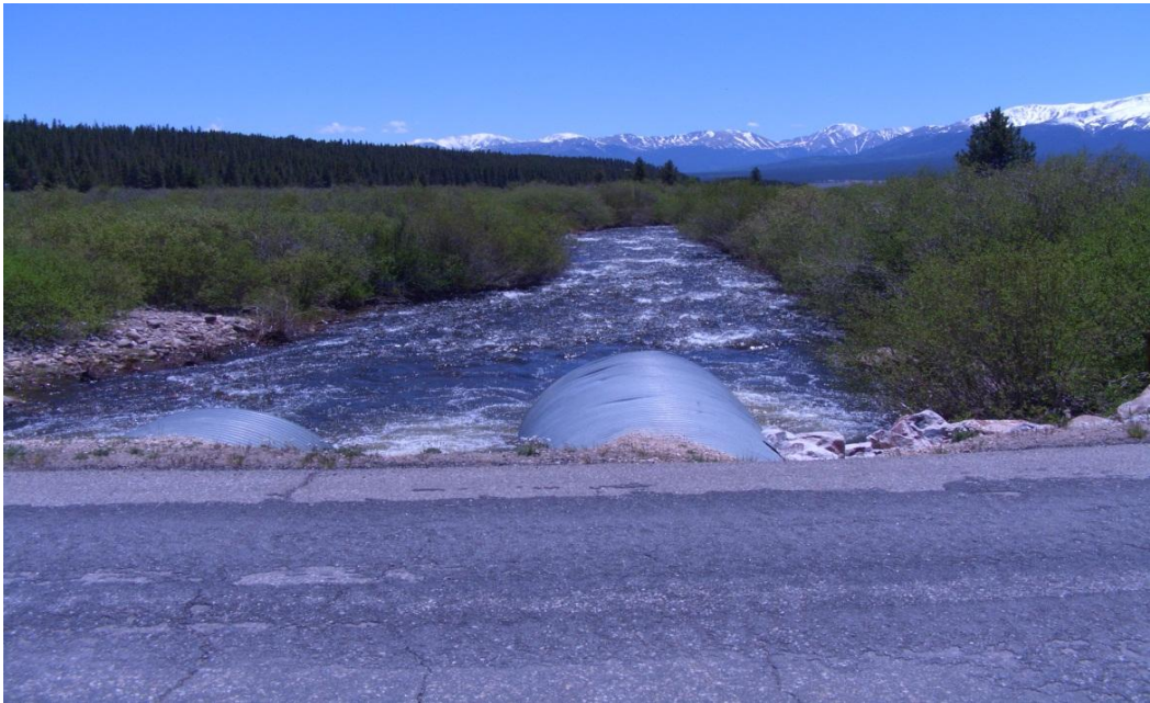
Figure C-62: County Road 4 bridge over Arkansas River, looking downstream (south).
