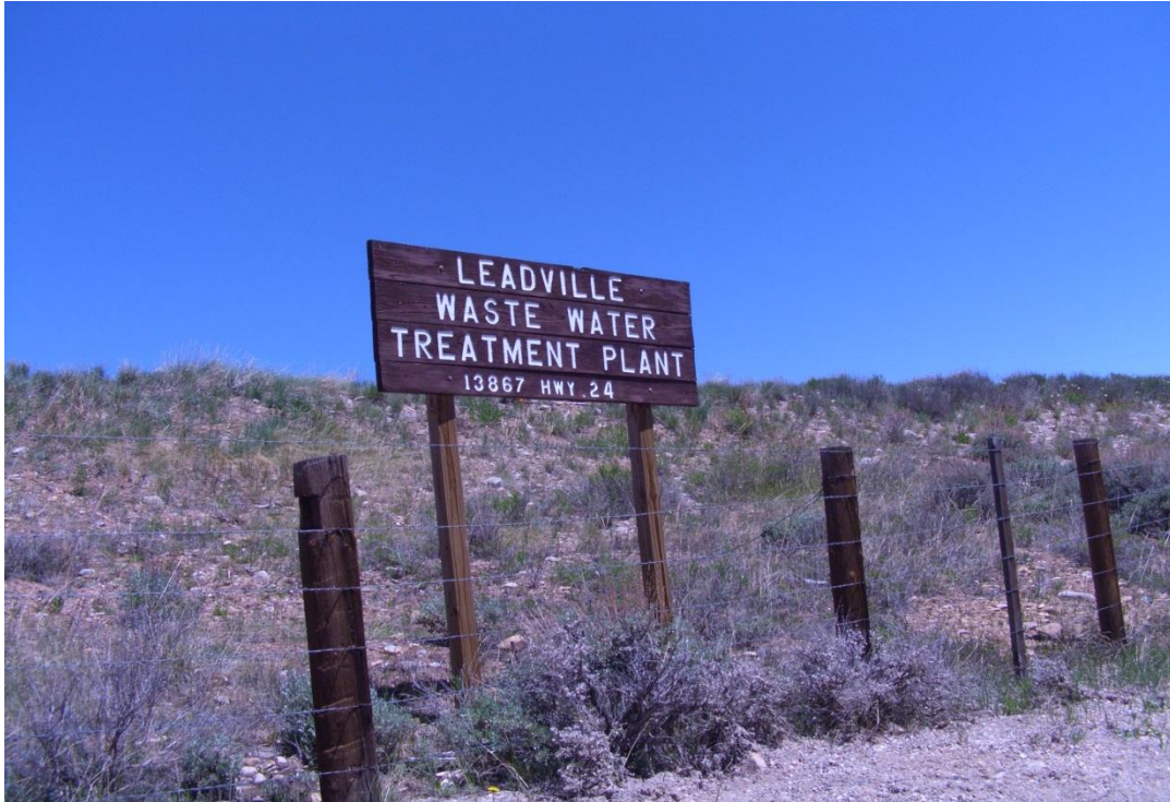
Figure C-43: Entrance to Leadville Waste Water Treatment Plant (WWTP).
