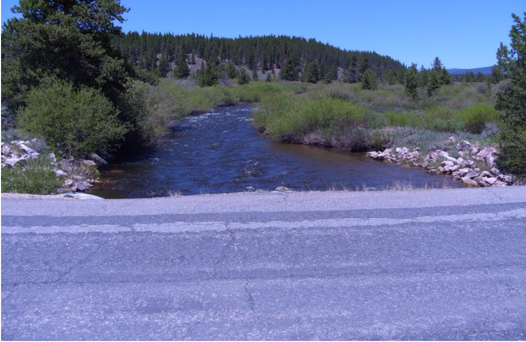
Figure C-61: County Road 4 bridge over Arkansas River, looking upstream (north).
