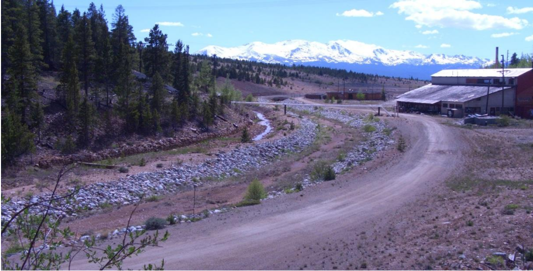
Figure C-9: View down California Gulch below Yak Tunnel Portal. Channel transmits flow to Yak Water Treatment Plant. Right channel is the California Gulch drainage.
