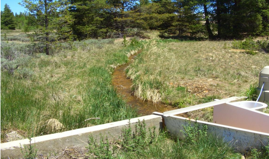
Figure C-32: View upstream from right bank at CG-5 flume.
