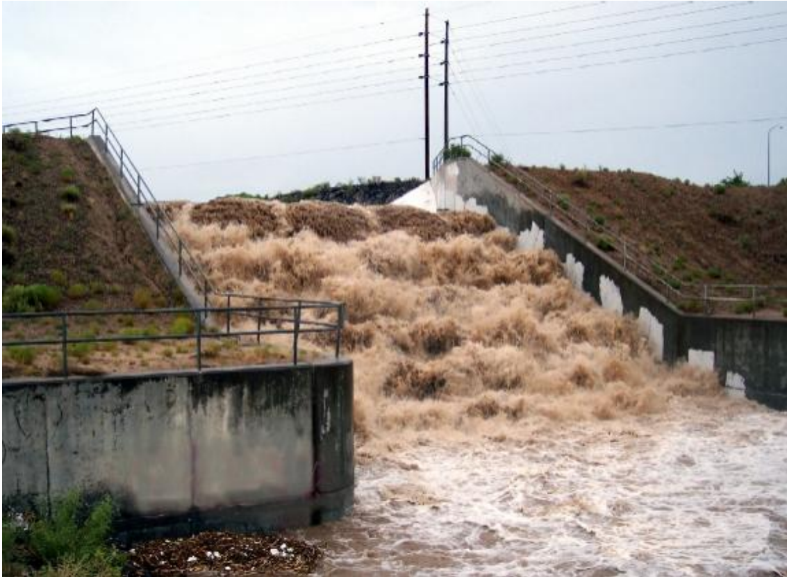
Figure 4.14 - Steep drop in a storm drainage channel (from AMAFCA)
