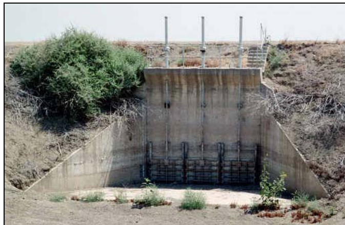
Figure 8: Evacuation Culvert Located in Sediment Basin near Railroad
