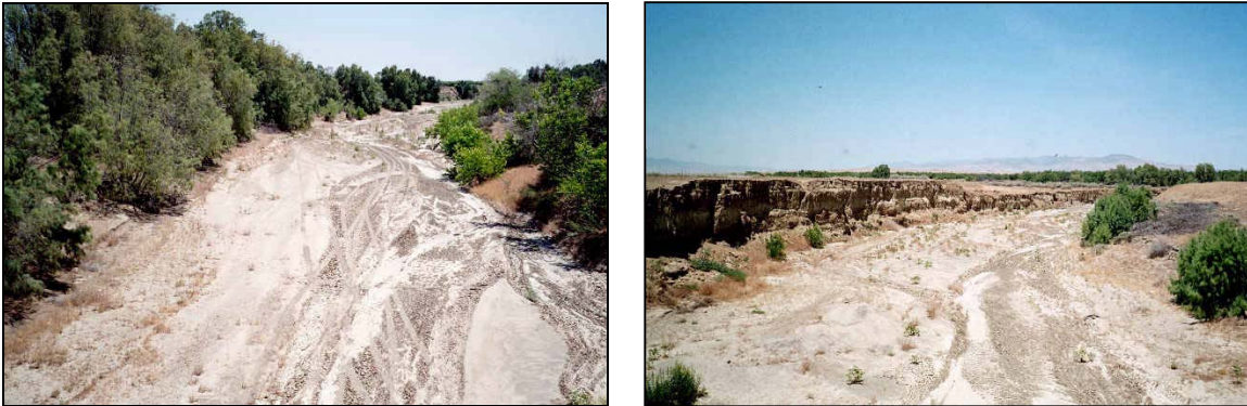
Figure 3: El Dorado Avenue Looking Downstream and Upstream
