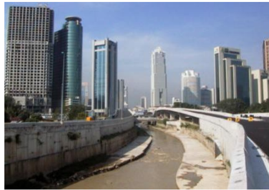
d) Flood wall along the channel
