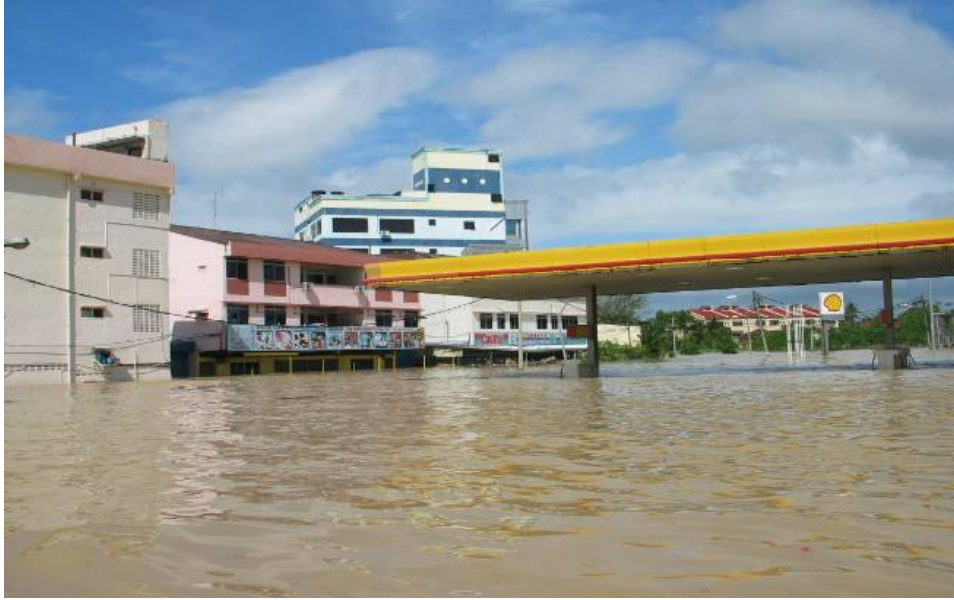
Figure 5.7: Gas station could be exposed to the risk of fire from flood pressure
