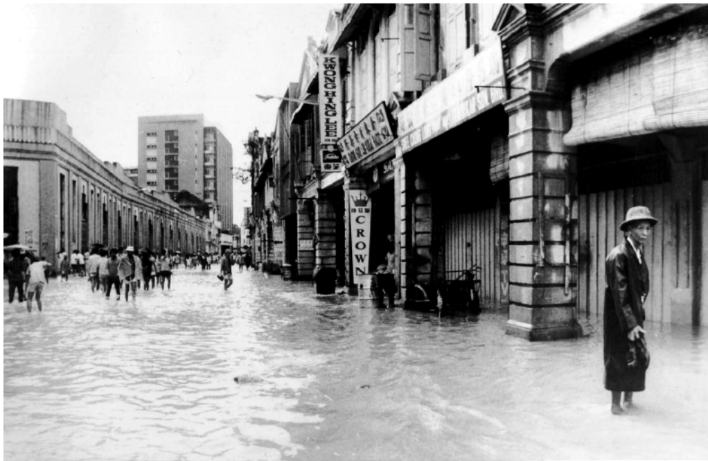
Figure 6.2: Kuala Lumpur Flood of 1971 (DID)
