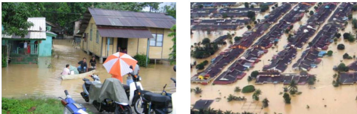
Figure 6.13: Flood impact in elevated houses and modern houses (DID, 2007)
