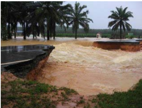
c) Public cleared the unstable ground
