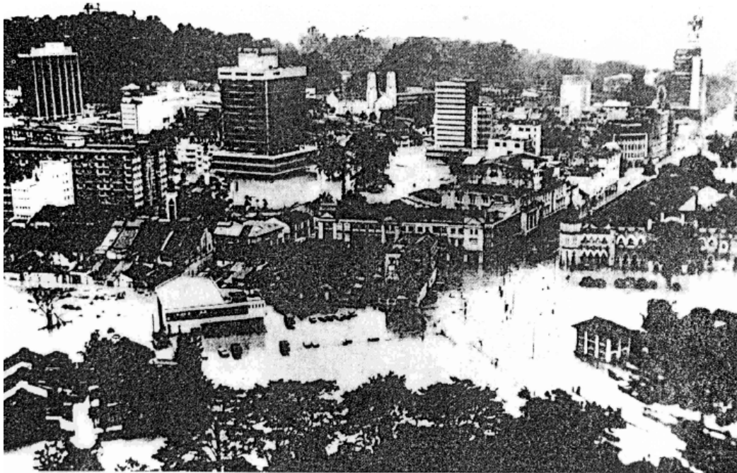
Figure 6.1: Kuala Lumpur Flood of 1971 (DID)
