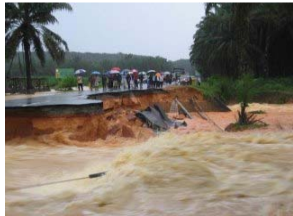
b) Cutting through the road
