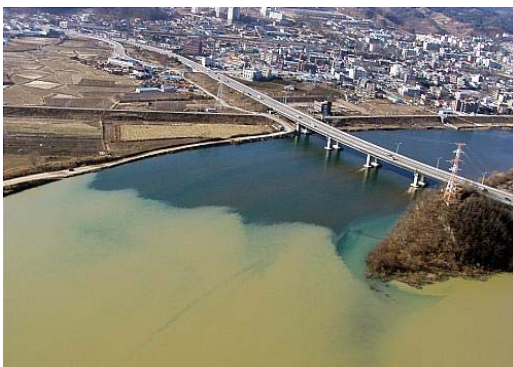
(a) Downstream of Soyang Reservoir (2006)
