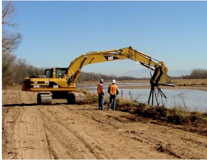
Fig. 17: Los Lunas, west bank. The first day of jetty jack removal, Apr. 9, 2002. Bankline jacks are the first to be removed. The job of removing 1,355 jacks is expected to take one to several months. Photo by Mark Horner, U.S. Army Corps of Engineers.
