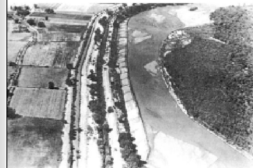
Fig. 9(b): Jetty field installed. Photo: Aug. 12, 1953.
