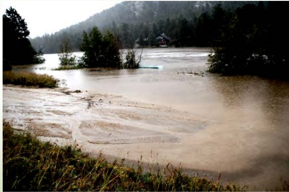
Rainbow Lake just before dam failure
