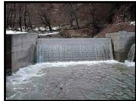
Precast Concrete Weir
