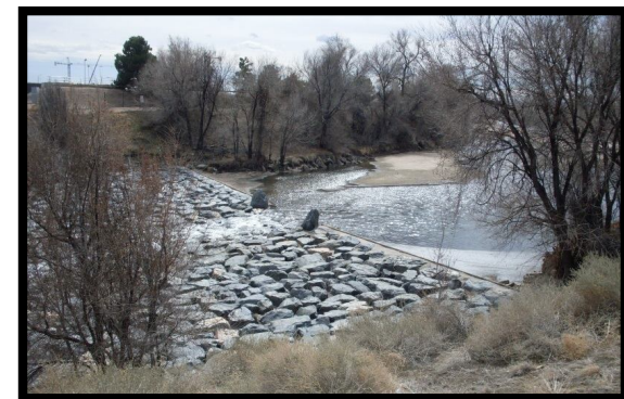
Sloping Grouted Boulder Drop
