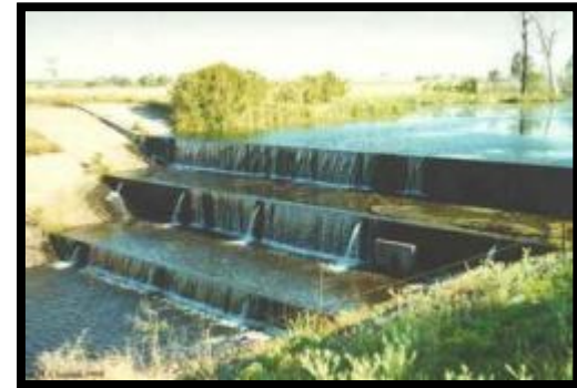
Steel Sheet-Pile Weir
