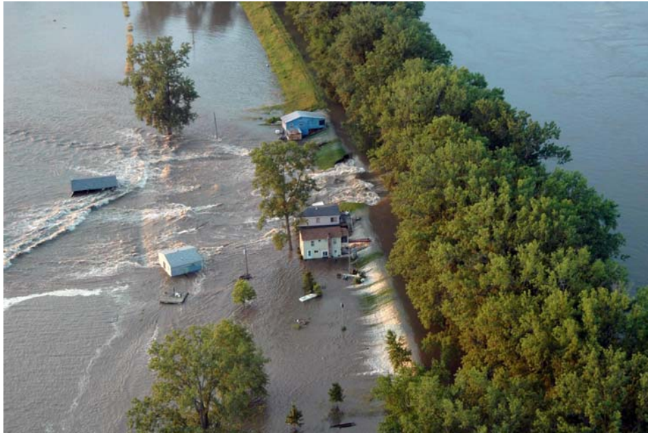
Figure 12. Winfield-Pin Oak breach (USACE St. Louis District 2008).
