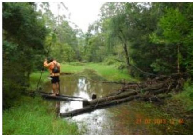
Photo b. Constructed bed control large wood structure in Australia (Andrew Brooks).
