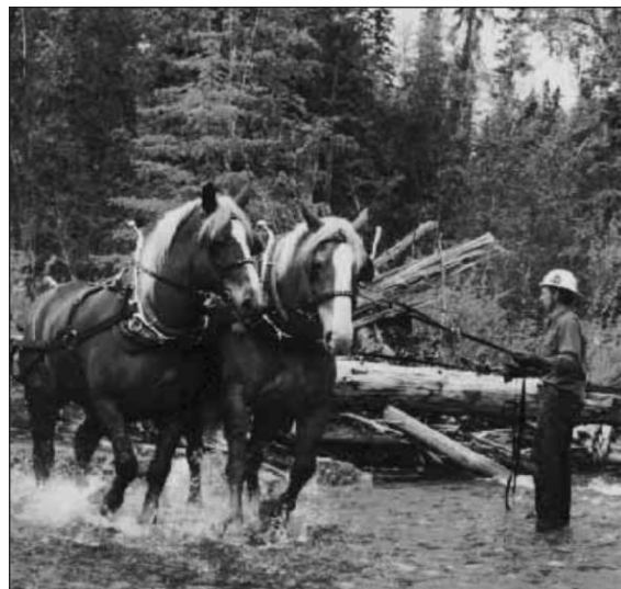
Figure 8-10. Belgian Draft Horses Moving Large Wood for Instream Placement
