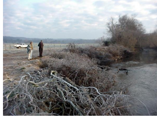
Photo h. Large wood with complex fine branches placed along outside of bend to trigger sediment deposition along steep, eroding bank of a Georgia stream.
