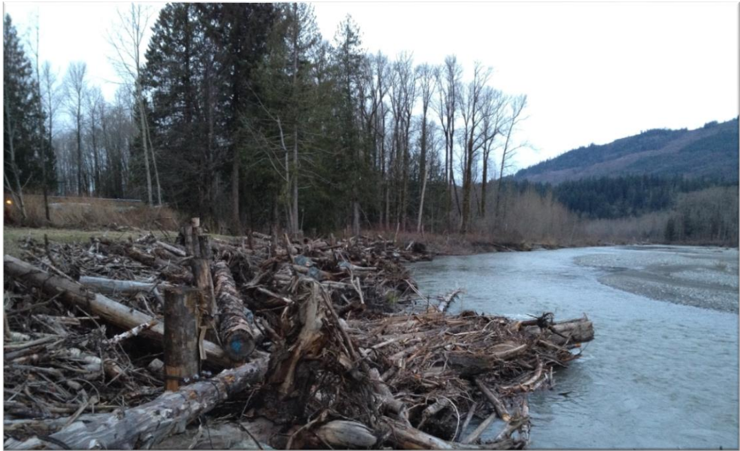
Complex timber revetment designed to protect bank by partitioning shear stress while also creating cover and hydraulic refugia for salmonids, South Fork Nooksack River, Northwest Washington (Tim Abbe 2012)
