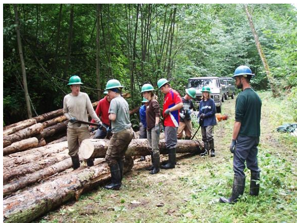
Figure 8-9. Manual Labor Team Stockpiling Large Wood Prior to Stream Installation
