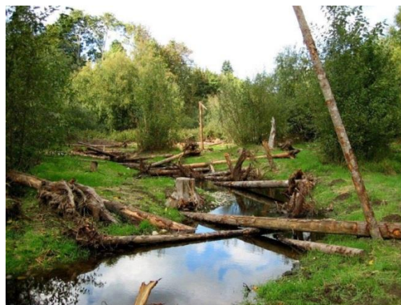
Figure 6-14. Entanglement of Logs in Riparian Stumps and Boles for Passive Restraint, Hylebos Creek, Milton, Washington
