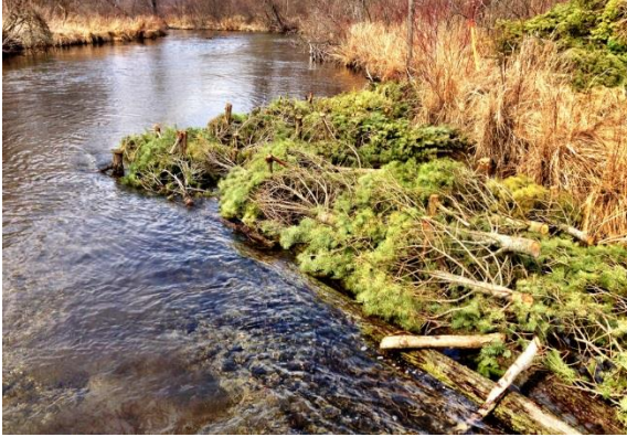
Photo g. Wood structure placed to accelerate flows and flush fine sediment deposited on gravel bed of Fawn River, Ohio, following rapid drawdown of an upstream impoundment. (Photo courtesy of Fawn River Restoration and Conservation Charitable Trust.)
