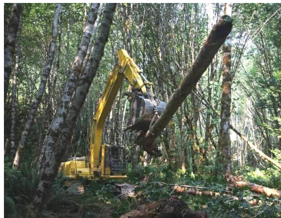
(a) Use of excavator with bucket and hydraulic thumb to position log with rootwad. (b) Use of rotating grapple to move multiple small logs. (c) Log tongs used to position rootwad log in tight quarters.
