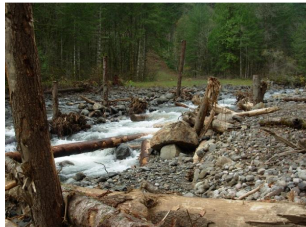
Figure 2-3. Woodward Creek Pipeline Crossing Wood Placement, Washington
