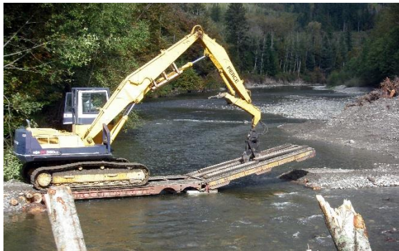
Figure 8-5. Examples of Temporary Bridges Constructed for Large Wood Projects
