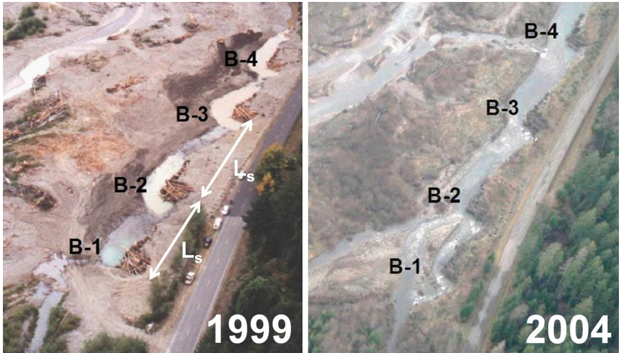
Figure 6-7. ELJ Spacing to Protect Road and Enhance Habitat Along the Cispus River
