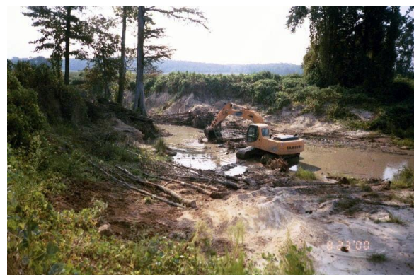
Figure 8-6. Minimal Excavation for Placing First Layer of Large Wood
