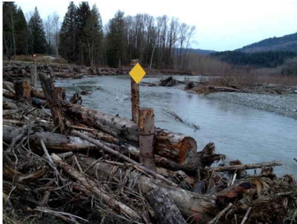
Figure 2-6. A Warning Sign on Wood Placement, South Fork Nooksack River, Washington
