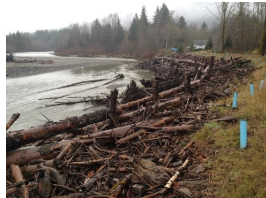
Photo d. Complex timber revetment with internal rock collar ballast, 2010 (Tim Abbe).
