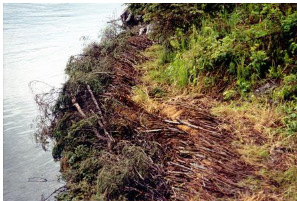
Figure 6-6. Continuous and Intermittent, Spur-Type Large Wood Structures
