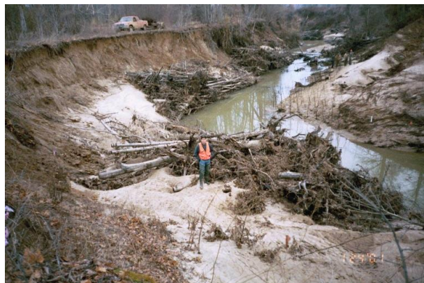
Figure 6-6. Continuous and Intermittent, Spur-Type Large Wood Structures
