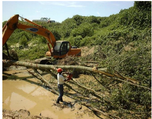
Figure 8-1. Use of Locally Sourced Large Wood
