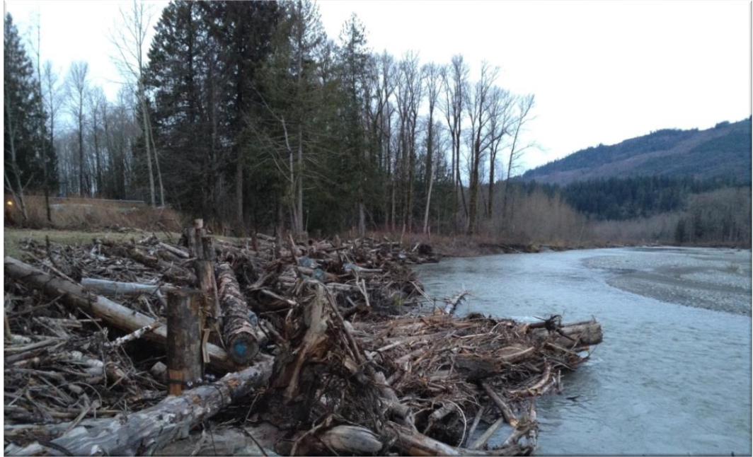
Complex timber revetment along South Fork Nooksack River, Washington (Tim Abbe 2012)
