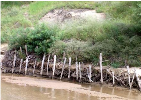
Photo a. Bundles of small wood have been used for several thousand years in China to stabilize banks and levees (Glenn Wilson).
