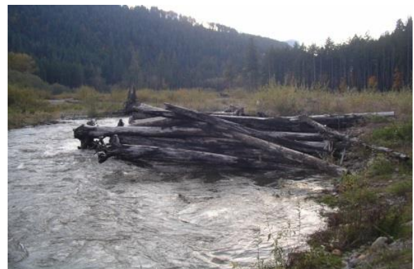
Photo f. Detail of engineered logjam, Cispus River, Washington, 2004 (Tim Abbe).
