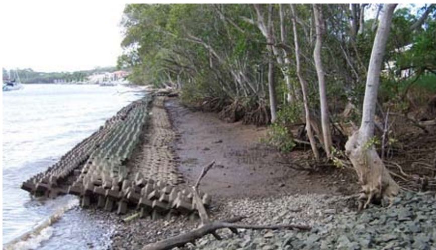
Figure 6. A-Jacks revetment at Charles Holm Park.
