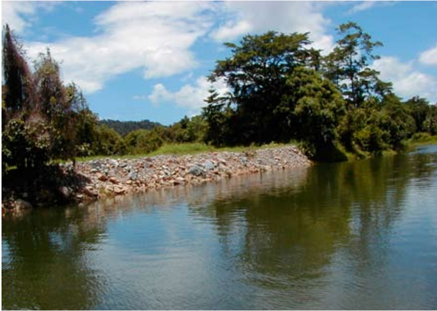
Figure 3. Rock revetment, Russell River.
