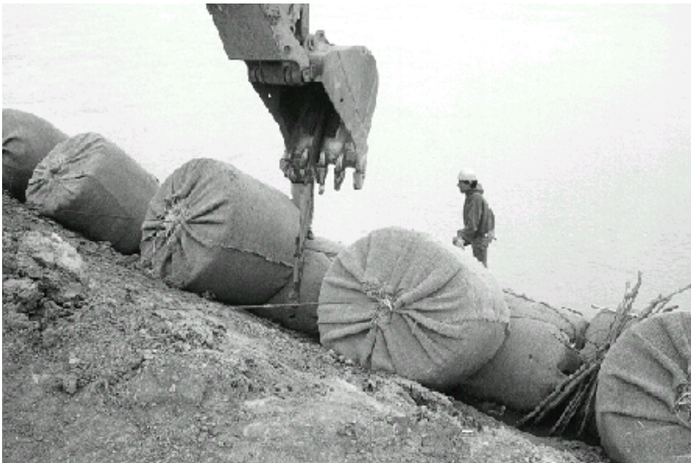
Figure 5.35. Backhoe digs bigger diameters
