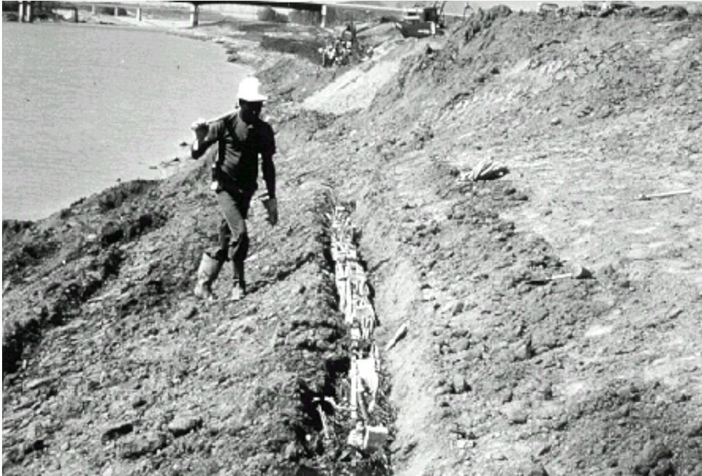
Figure 5.39. Installing contour wattling
