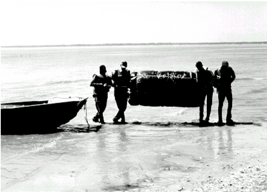
5.24b. Coir fiber mats being carried to site
