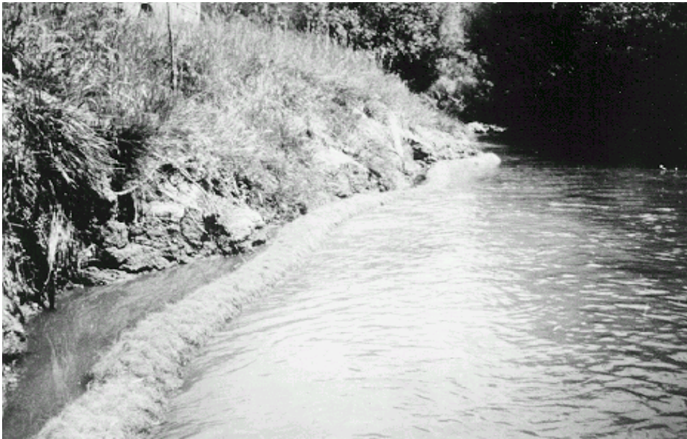
Figure 5.23a. Coir roll installed at stream edge (photo courtesy of Bestmann GmbH, Wedel, Germany)
