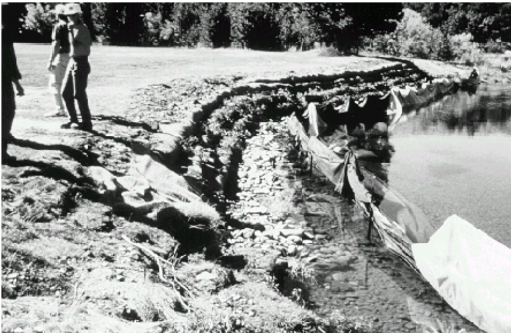
Figure 5.31. Upper Truckee River site before construction
