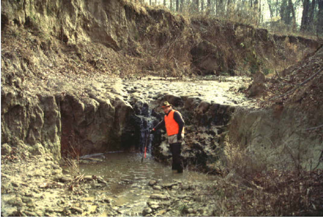
Figure 3.22 Knickpoint in a Degrading Channel
