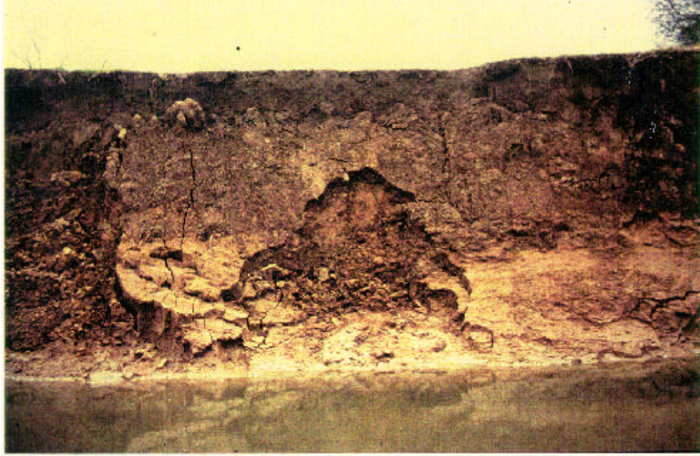
Figure 3.35 Pop-out Failure
