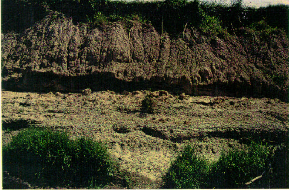
Figure 3.26 Erosion Generated by Piping
