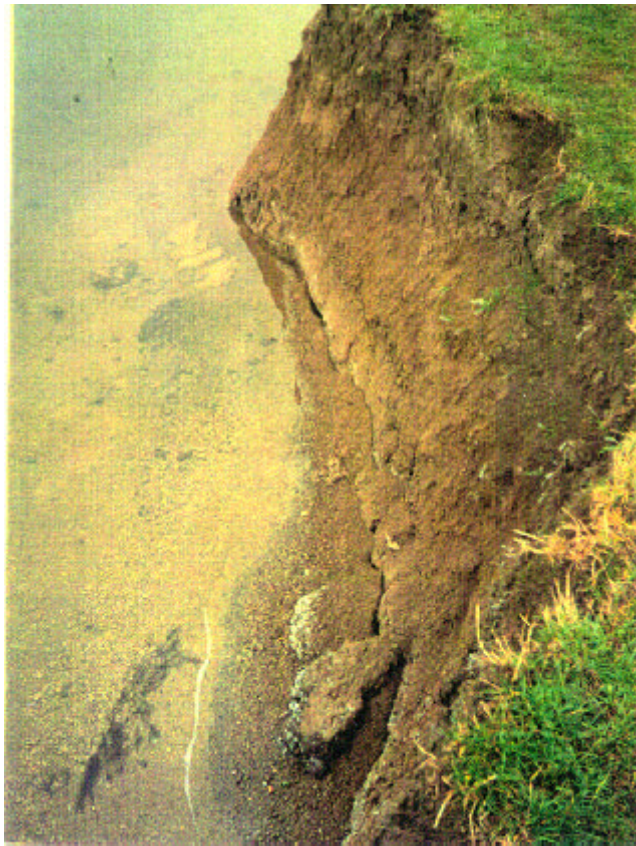
Figure 3.27 Erosion Generated by Freeze/Thaw
