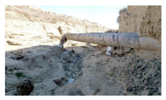
Figure 9.—Formerly buried pipeline exposed by gully incision (note headcut in lower left) in a desert wash, Navajo Reservation, New Mexico. Photo: Michael Sixta, Reclamation.
