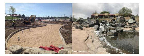
Figure 12.—Left: A sand and gravel filter was used to clean urban stormwater from a parking lot along the South Platte River near Denver, Colorado. Right: Stormwater and tributary baseflow are discharged through a scenic grade control and energy dissipation structure just before entering the South Platte River in Denver, Colorado. Photos: Tim Randle, Reclamation.
