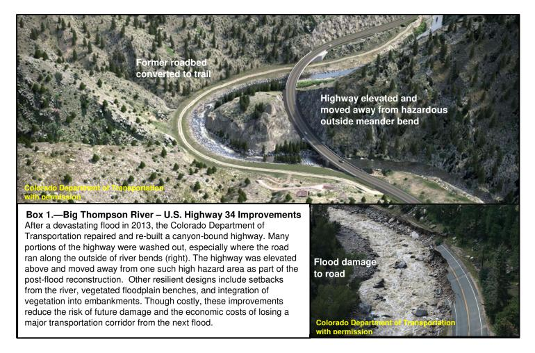
replaced or repaired, compatibility with the stream environment should be considered along stream and floodplain rehabilitation options to mitigate impacts. Managing riverine infrastructure within the context of master plans that account for watershed-scale processes and environmental concerns can result in proactive and more resilient, rather than reactive, infrastructure programs.
