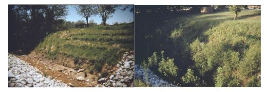
Figure 11.—Example of streambank bioengineering (right side of pictures) with riprapped bank (left side of pictures) in first year of construction (left) and two years later (right). Credit: Natural Resources Conservation Service.
