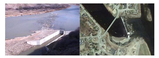
Figure 15.—Left: A low-head diversion weir constructed from natural, non-grouted materials replaced a push-up dam on the North Fork of the Gunnison River, Colorado. It allows for fish and boater passage and provides a low-maintenance solution for water diversion. Right: A bypass channel constructed around Howland Dam, Maine, for migratory fishes. Photos: Jeff Crane, Crane and Associates, Inc. (left) and Google Earth (right).
