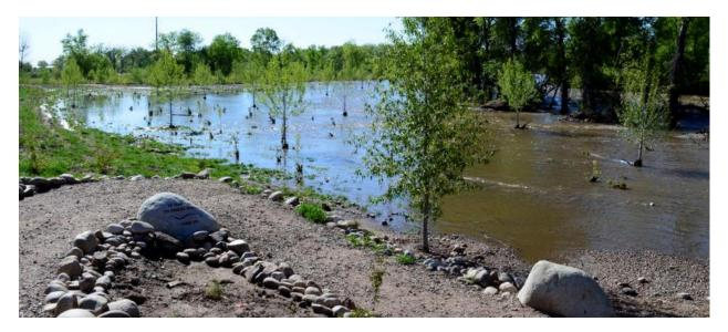
Figure 7.—Example of a floodplain rehabilitation on the Poudre River, Fort Collins, Colorado. A levee was removed and a floodplain bench excavated and revegetated to hydrologically connect with the incised river. Gravel quarries adjacent to the river were also reclaimed and connected with flood flow paths. Photo: Joel Sholtes, Reclamation.
