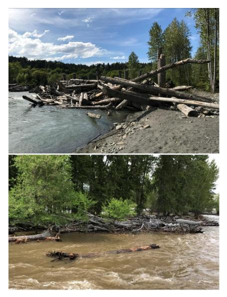
Figure 8.—Top: A pile-supported engineered log jam can increase water surface elevation immediately upstream, creating a pool for aquatic species, influencing the distribution of shear stress in Elwha River, Washington. Photo: Jennifer Bountry, Reclamation. Bottom: Large wood accumulation on a mid-channel island during spring runoff on the Methow River, Washington. Photo: Reclamation.
